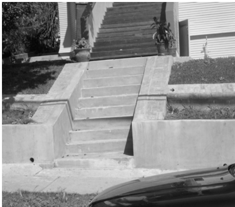
Historic retaining walls should be retained, repaired or replaced in-kind.
