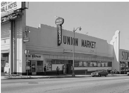
Others had flat roofs with decorative parapet detail, like this art deco market.
