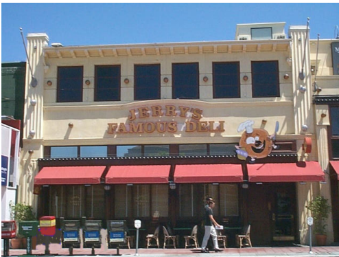
The parapet and other architectural details on this building help break up its physical bulk.
