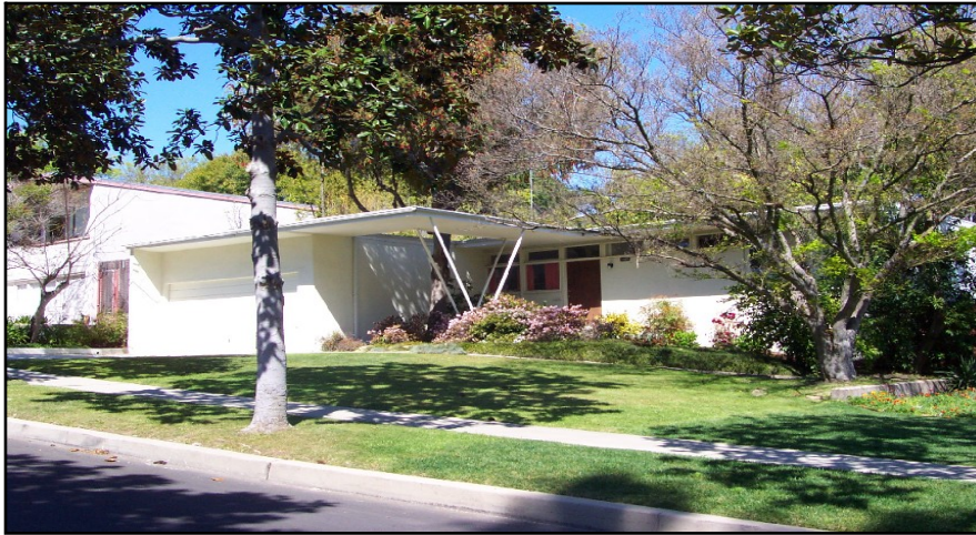
The Historic Context Statement will ground the survey's assessments within a comprehensive framework detailing Los Angeles' key property types, such as the post-World War II Modernist housing found in the Gregory Ain Mar Vista Tract HPOZ.
