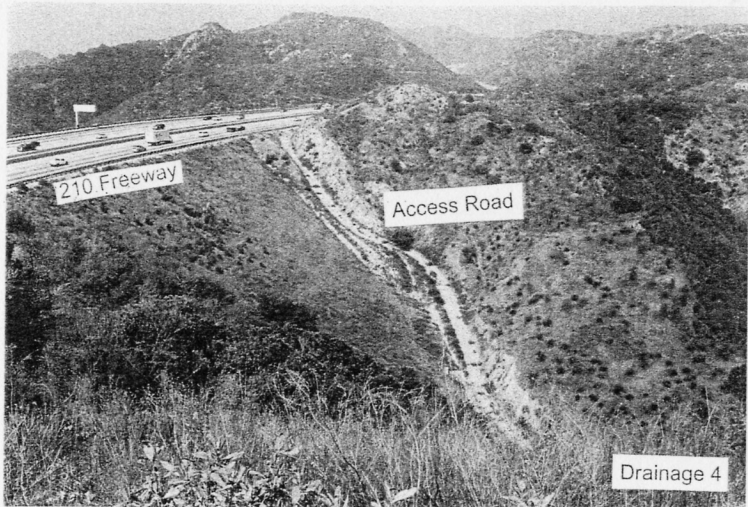
Photograph 9. View looking southwest at an access road connecting the 210 Freeway to Drainage 4. Coyote scat was detected within 10 meters of the 210 Freeway.
