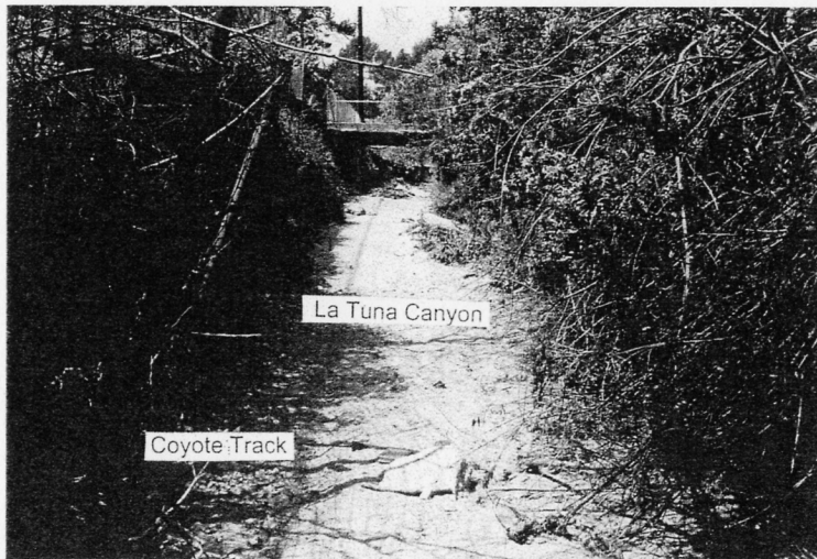
Photograph 33. View looking at La Tuna Canyon Wash off site, between property boundary and the La Tuna Canyon Was Debris Basin.
