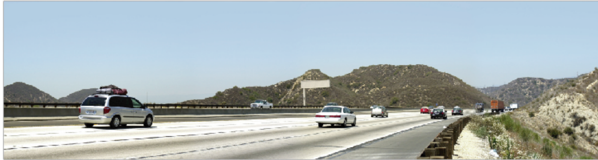
Existing view from the shoulders of Interstate 210 looking southwest toward proposed Development Area B.
