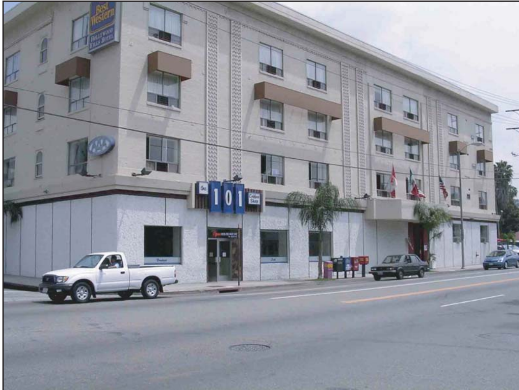
View 11: Looking northeast at the 4-story hotel opposite the project site on the north side of Franklin Avenue
