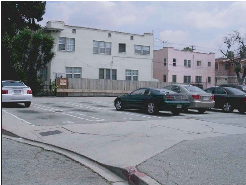
View 2: Looking northeast across the surface parking in the southern portion of the project site to the apartment buildings fronting onto Franklin Avenue
