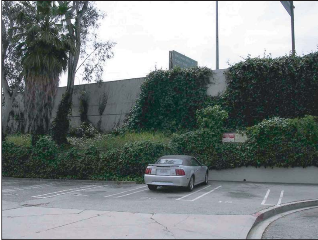
View 3: Looking south at the Hollywood Freeway (US 101) which borders the southern property line of the project site
