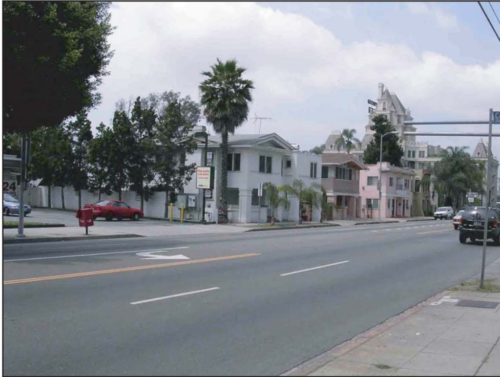
View 5: Looking southwest at the apartment buildings fronting onto Franklin Avenue in the northern portion of the project site
