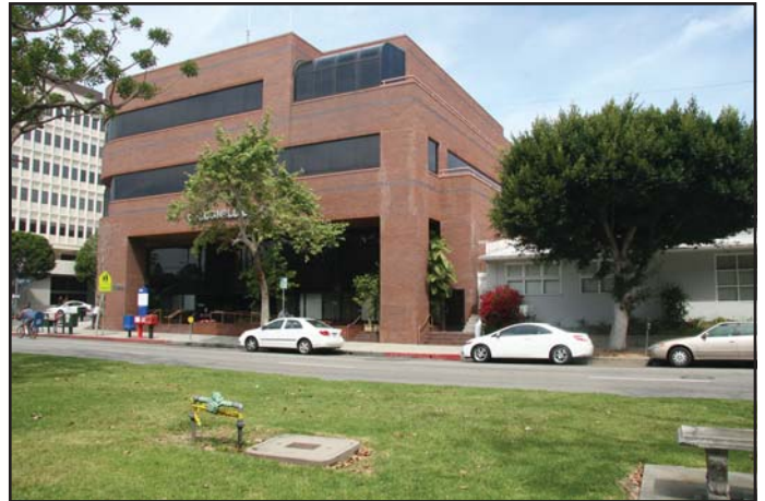
View 8: Facing northwest on San Vicente Boulevard view of southeastern facade of Coldwell Building, west of the project site.
