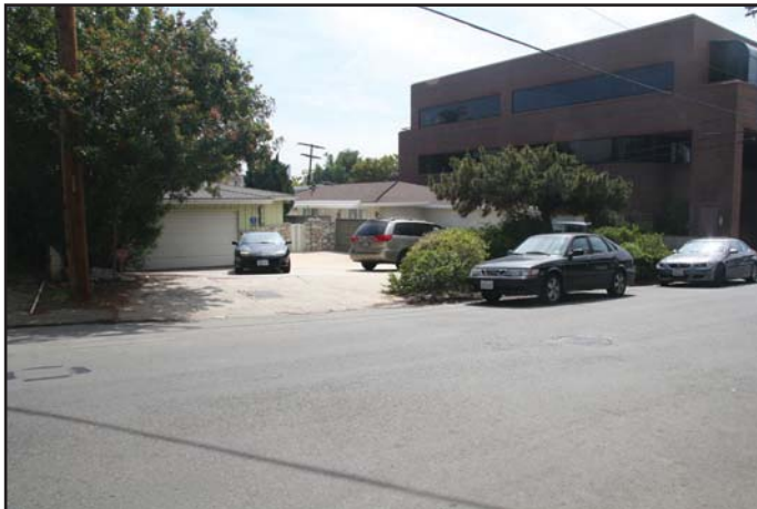
View 3: Facing southeast on Saltair Avenue, northwestern façade of residences at 644 and 642 Saltair Avenue.
