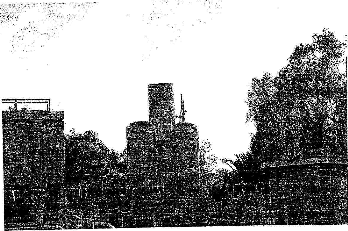
Vent Stack – where the oil and gas were vented to the air.
