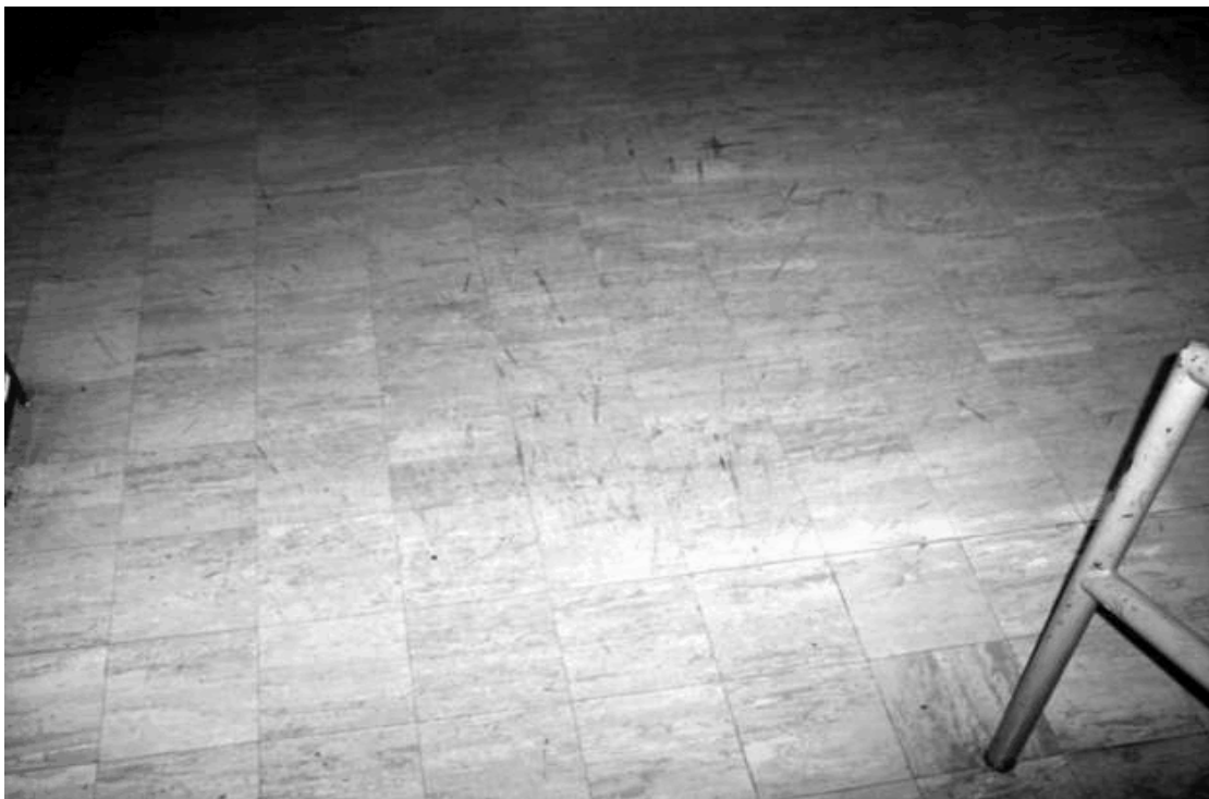
Typical Condition Of Floor Tile
