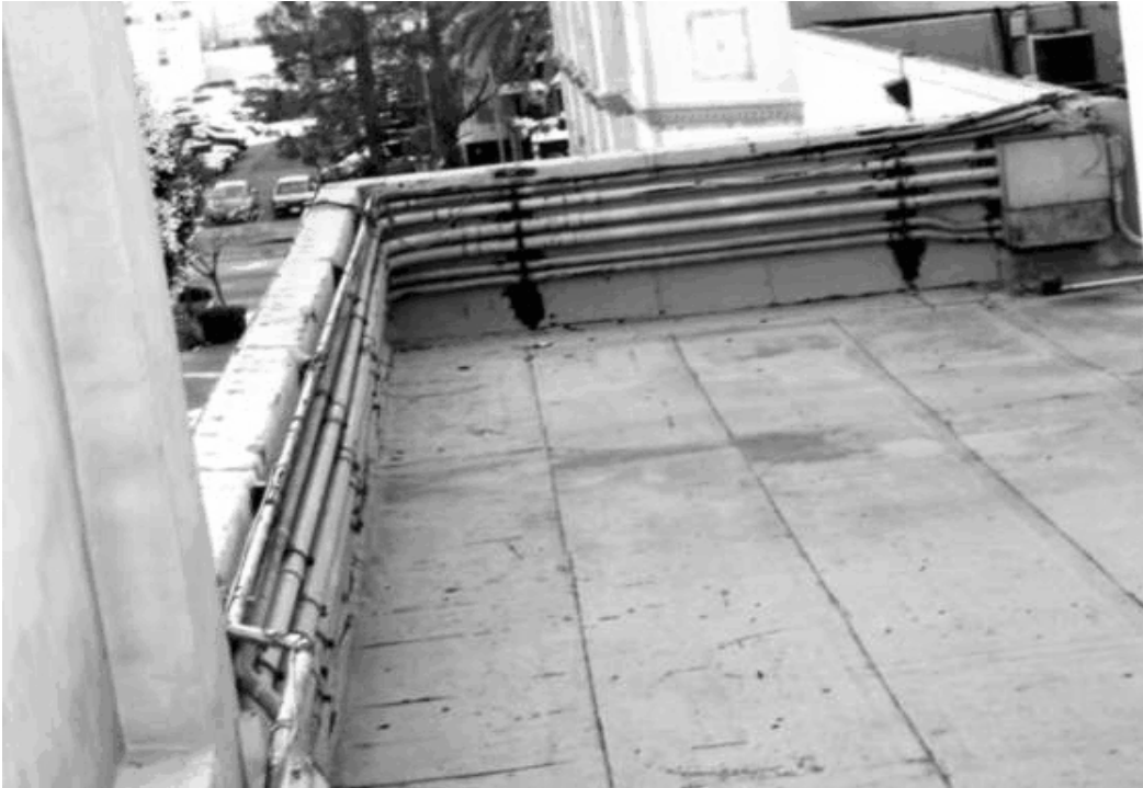
Typical Roofing And Mastic Material
