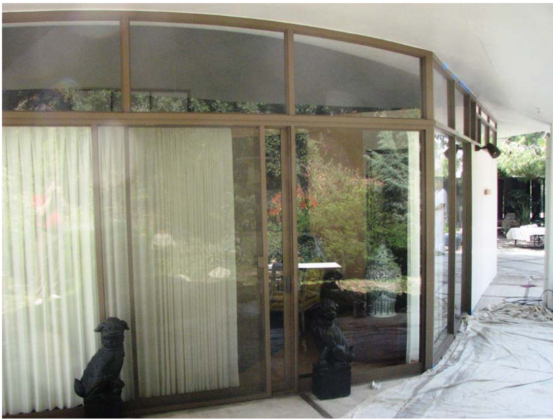
James F. Real Studio-Office, rear glass door, 77 Patrician Way (Photograph by Charles J. Fisher)
