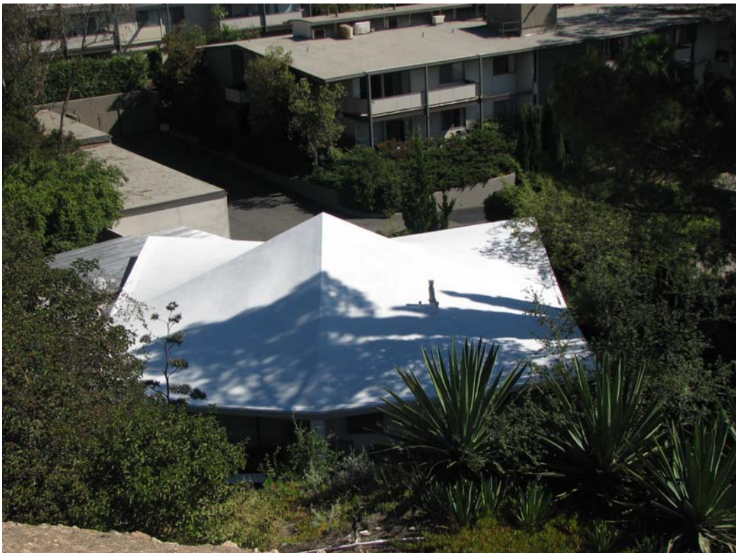
James F. Real Studio-Office, completed roof today, 77 Patrician Way (Photograph by Charles J. Fisher)
