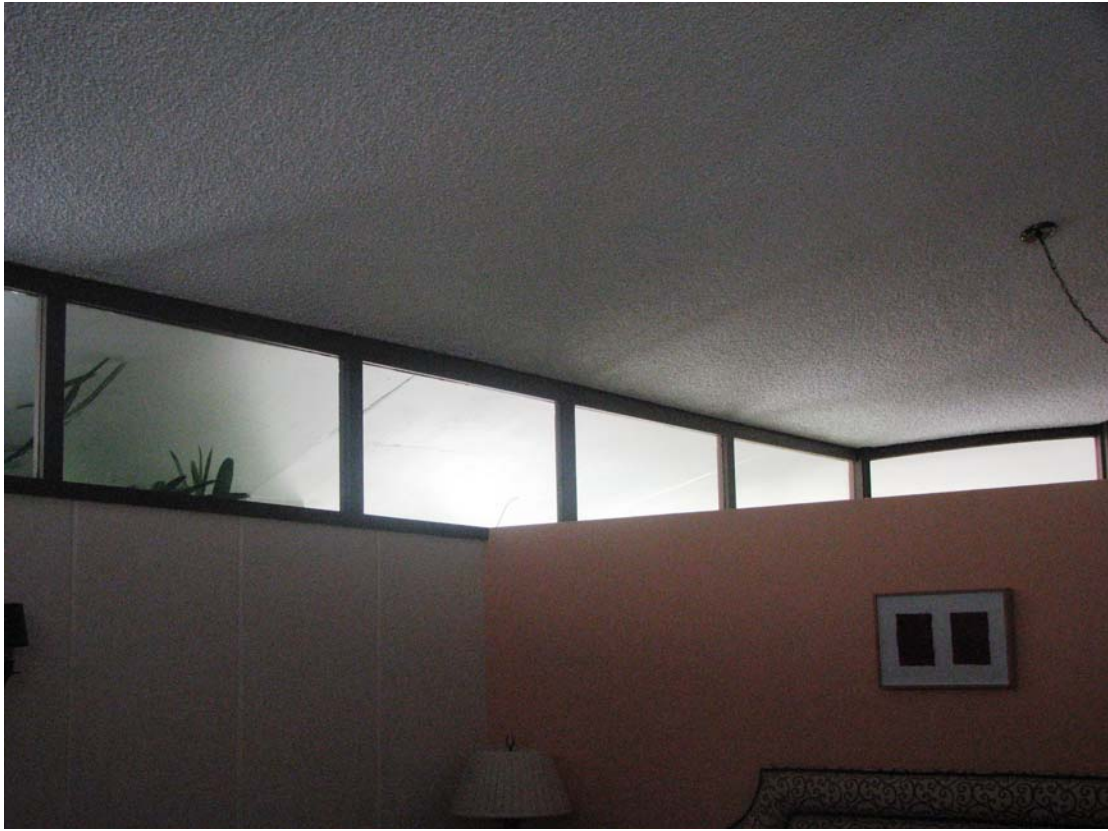
James F. Real Studio-Office, clerestory windows, 77 Patrician Way (Photograph by Charles J. Fisher)
