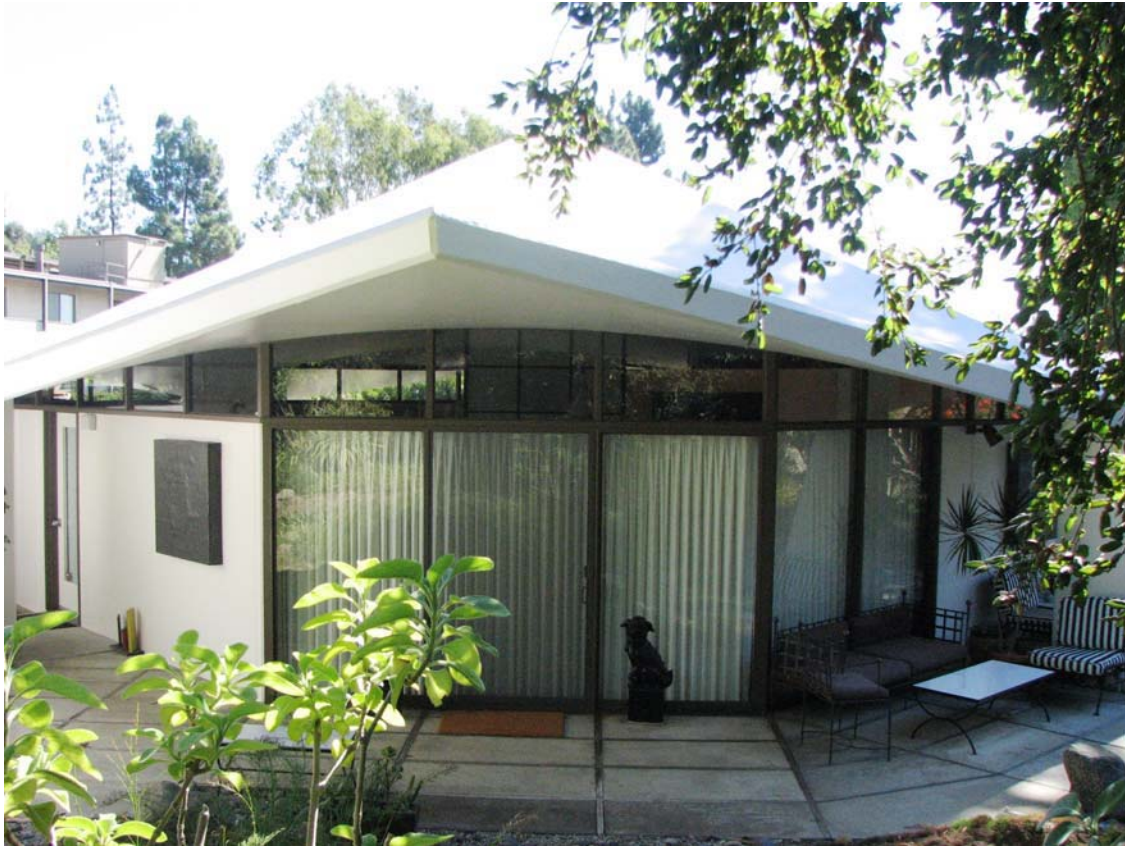
James F. Real Studio-Office, rear elevation, 77 Patrician Way (Photograph by Charles J. Fisher)
