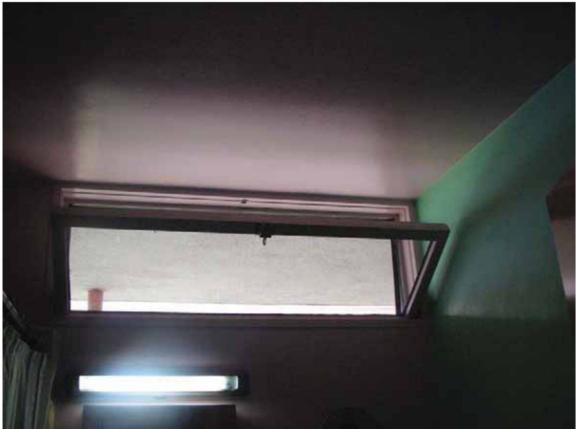
Henry Shire Residence, transom window, 2208 Princeton Avenue (Photograph by Charles J. Fisher)
