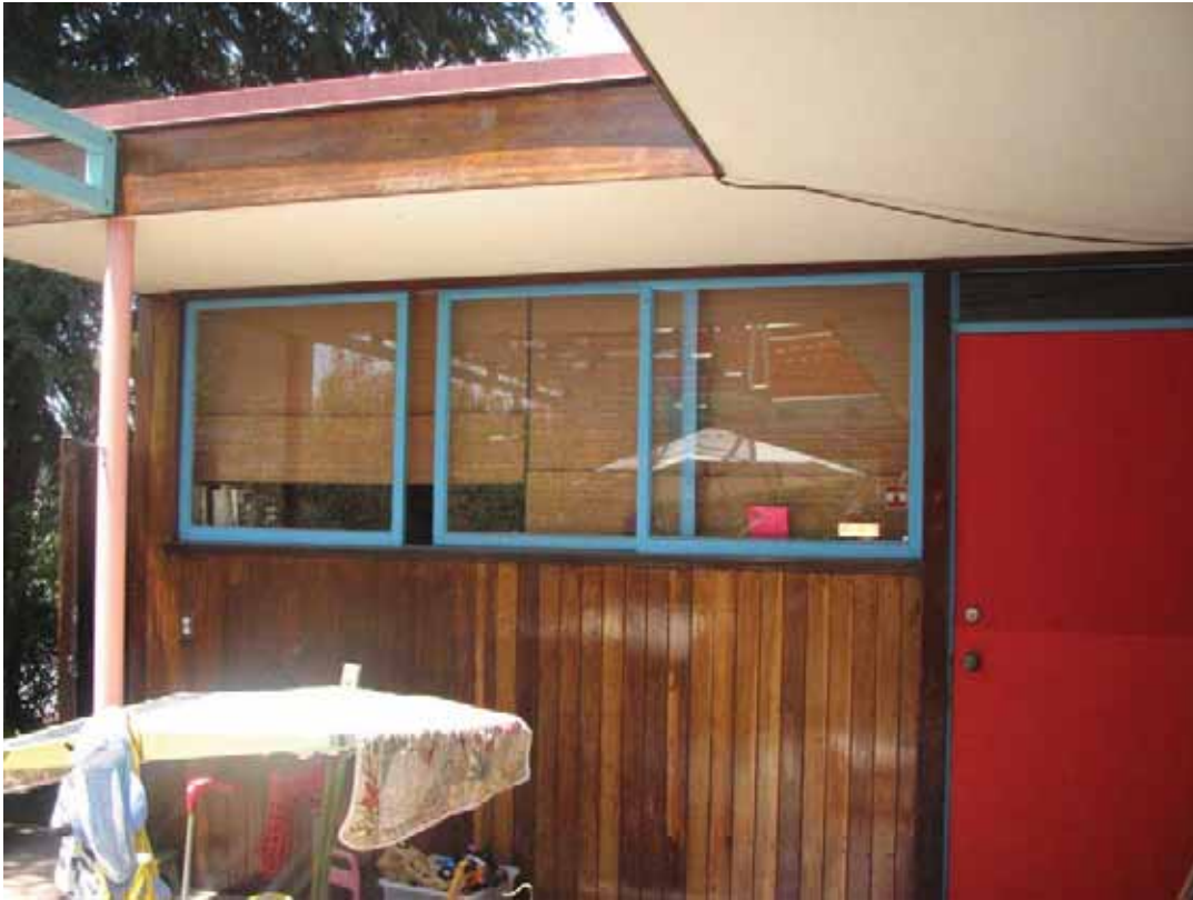
Henry Shire Residence, wood sliding window view from patio, 2208 Princeton Ave (Photograph by Charles J. Fisher)
