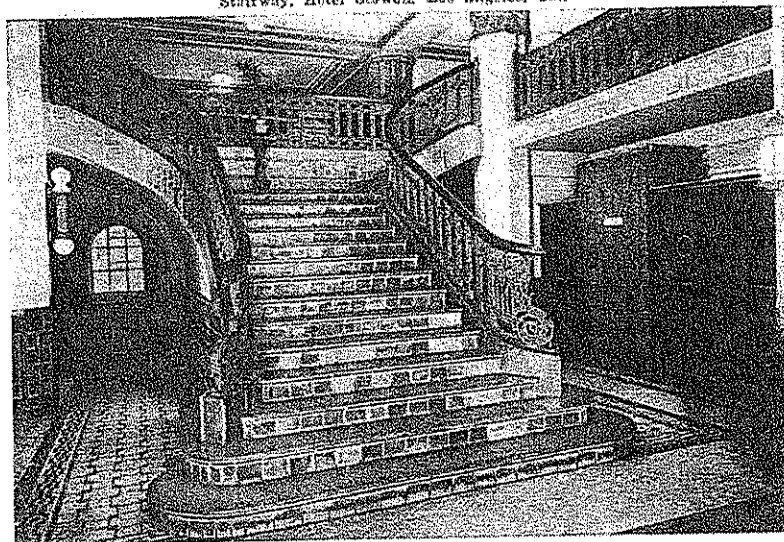
The grand stair in the lobby was cleaned and refinished. The plaster ceilings and the original tile are all intact today.
