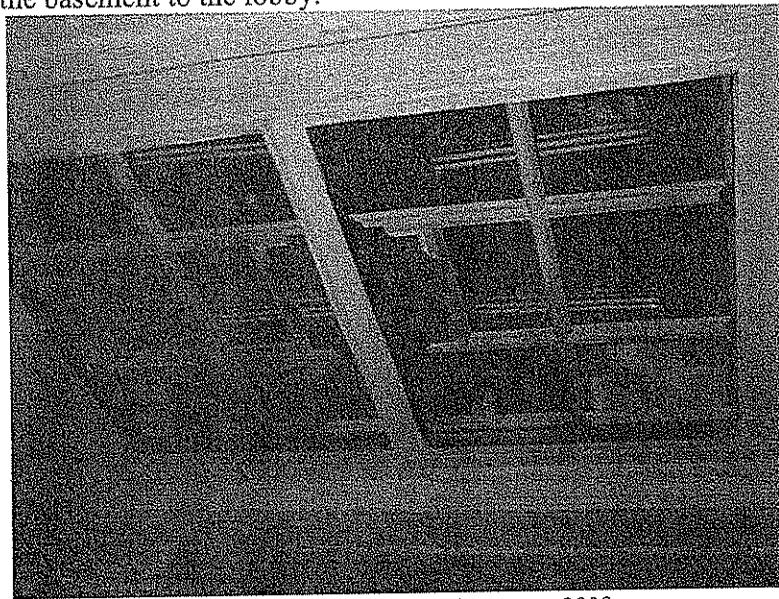
Skylights before the adaptive reuse, 2008
