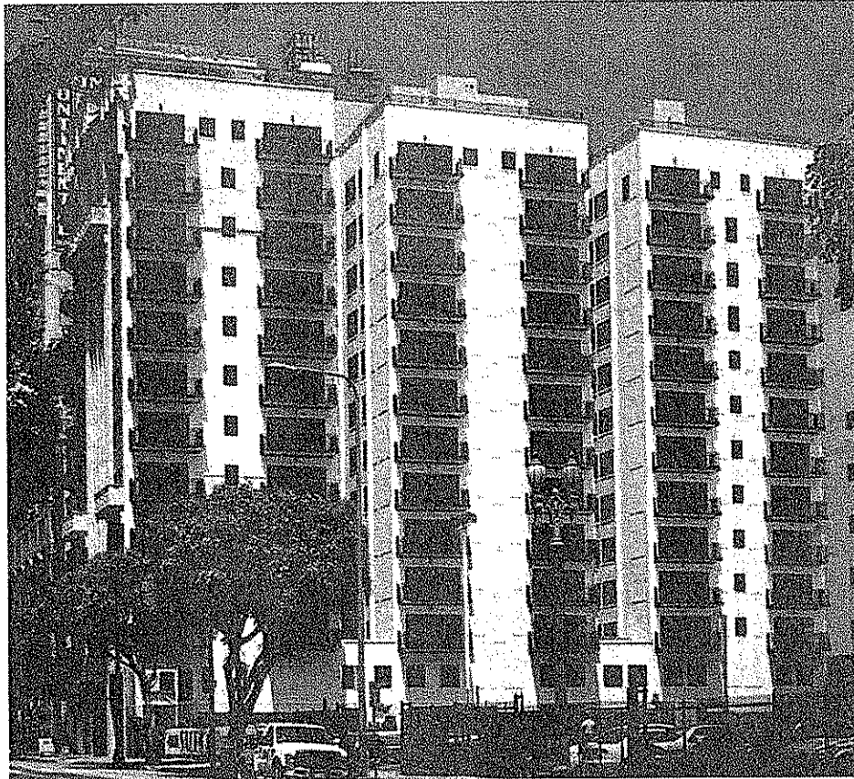
Before and After the Adaptive Reuse Project Note the fenestration pattern and the outlines / sills for sealed windows Source: Rockefeller Partners Architects
