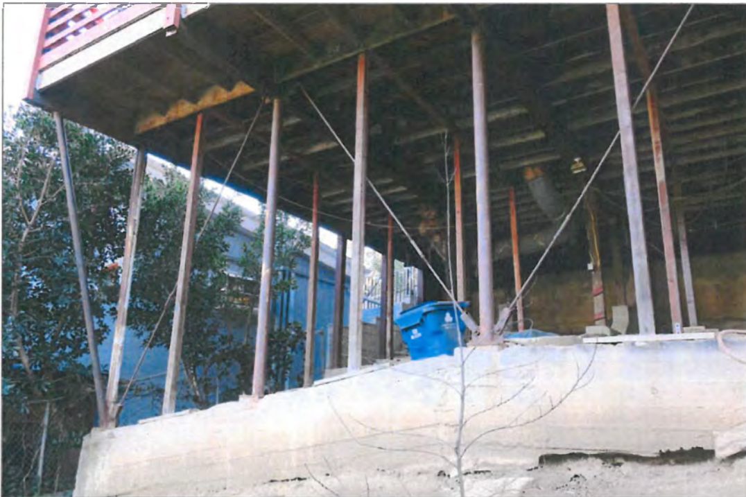
View of structural system beneath the house, view south (ARG, 2017).
