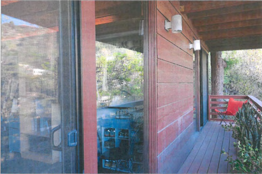
Detail of first floor deck, view west (ARG, 2017).
