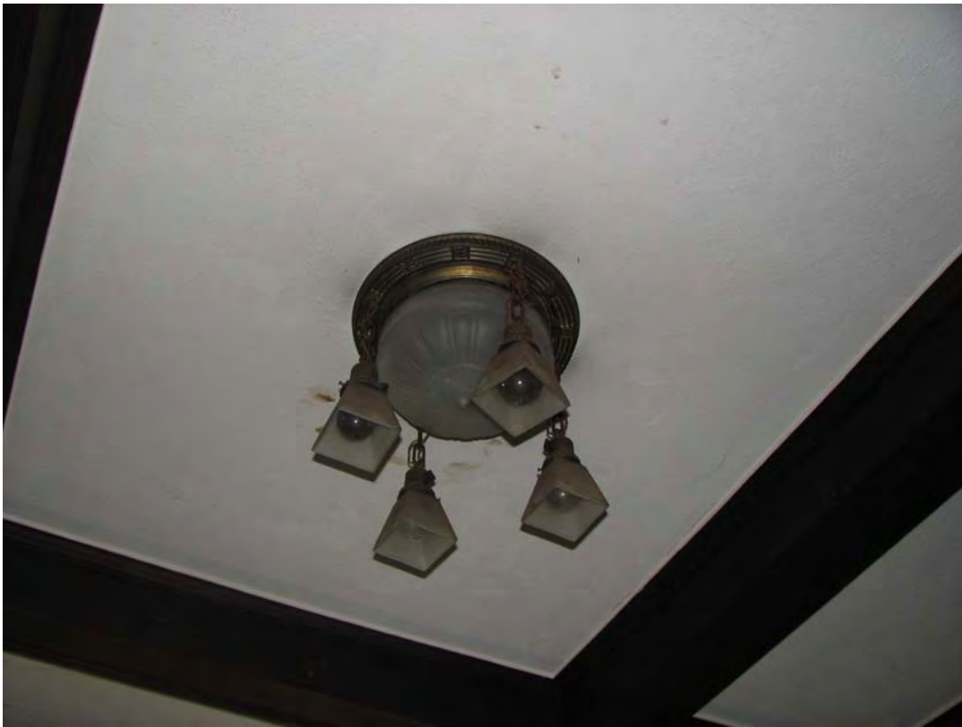
Young-Gribbling Residence, light fixture installed by Gribbling, 3320 Griffin Avenue, July 1, 2011 (Photograph by Charles J. Fisher)
