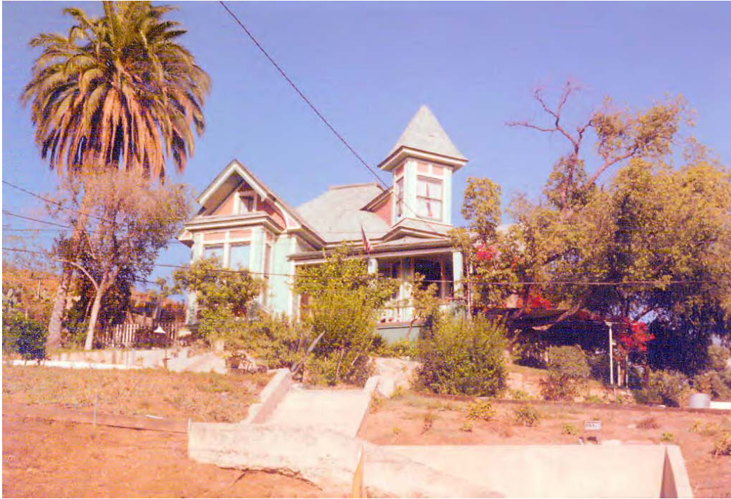
Young-Gribling Residence, 3320 Griffin Avenue, September 2, 1991 (Photograph by Charles J. Fisher)
