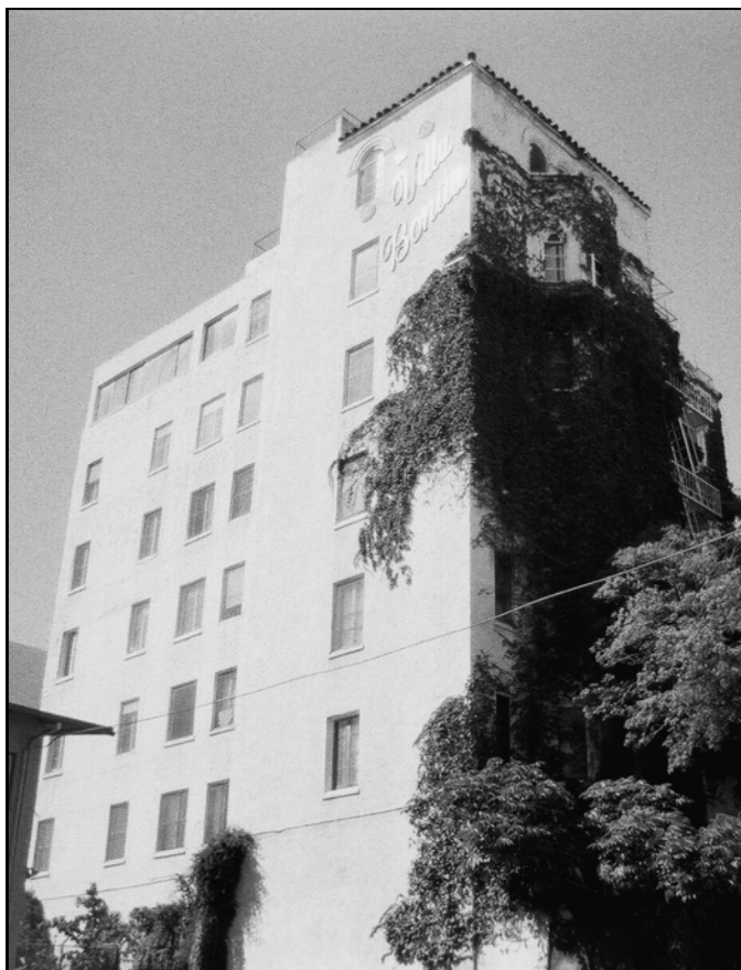
Photograph 1: Overall view northwest, south (left) and east (right) elevations (photo: Chattel Architecture, 2008)
