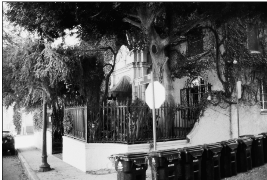
Photograph 5: Exterior view southwest, main entry fronting corner of Hillcrest Rd (left) and Bonita Terrace (right) (photo: Chattel Architecture, 2008)
