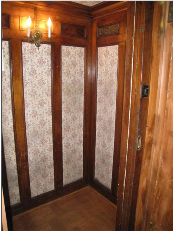
Photograph 9: Interior view, historic elevator cab (photo: Chattel Architecture, 2008)
