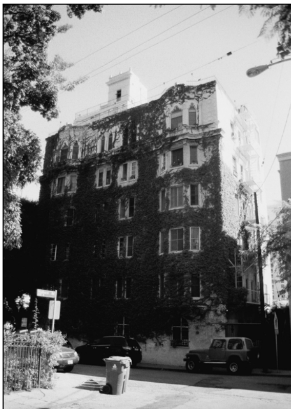
Photograph 6: Overall view southeast, north elevation fronting Bonita Terrace (photo: Chattel Architecture, 2008)
