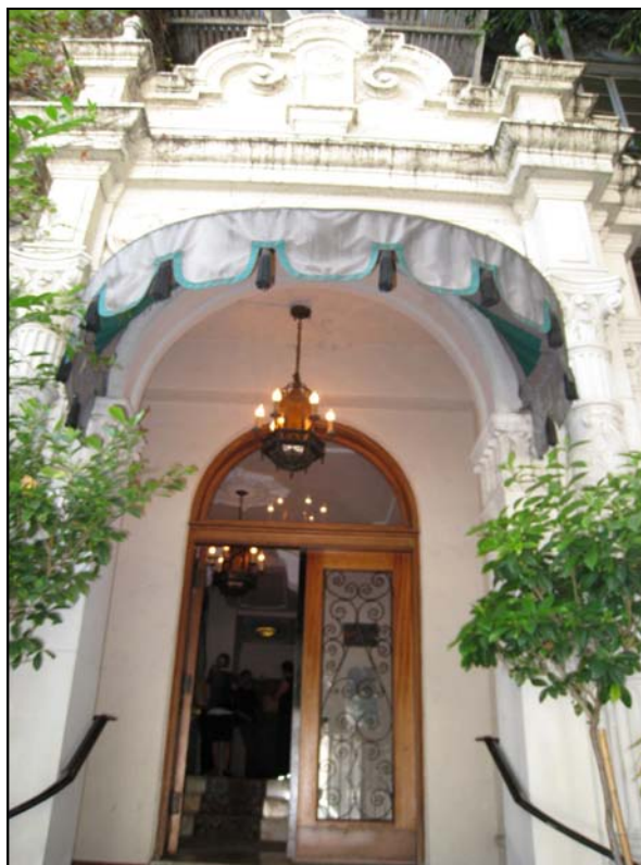
Photograph 7: View west, main entry on east elevation (photo: Chattel Architecture, 2008)
