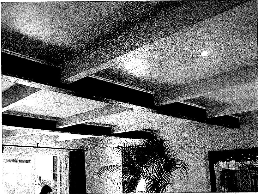
Kennedy-Solow House, living room ceiling, 6606 Maryland Drive (Charles J. Fisher photo)
