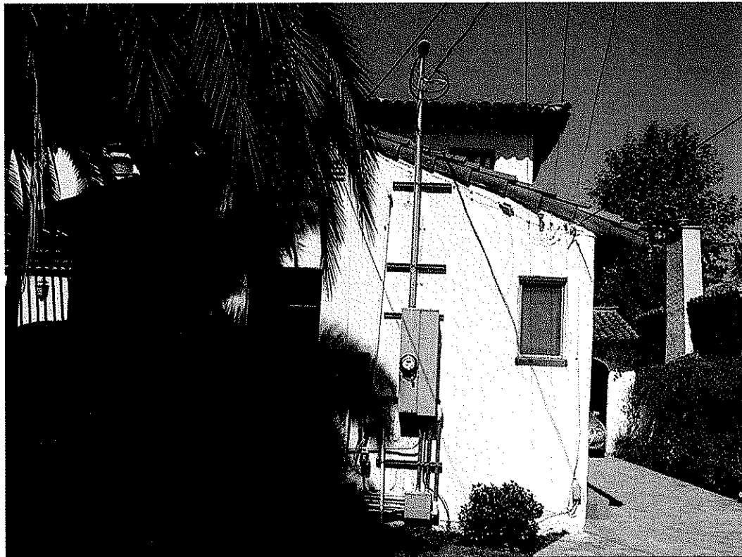
Kennedy-Solow House, rear elevation, 6606 Maryland Drive (Charles J. Fisher photo)
