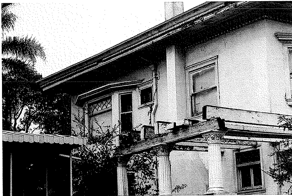
South elevation, bay window; chimney; and pergola, viewed to northwest. (Metal work is on neighbor's property).
