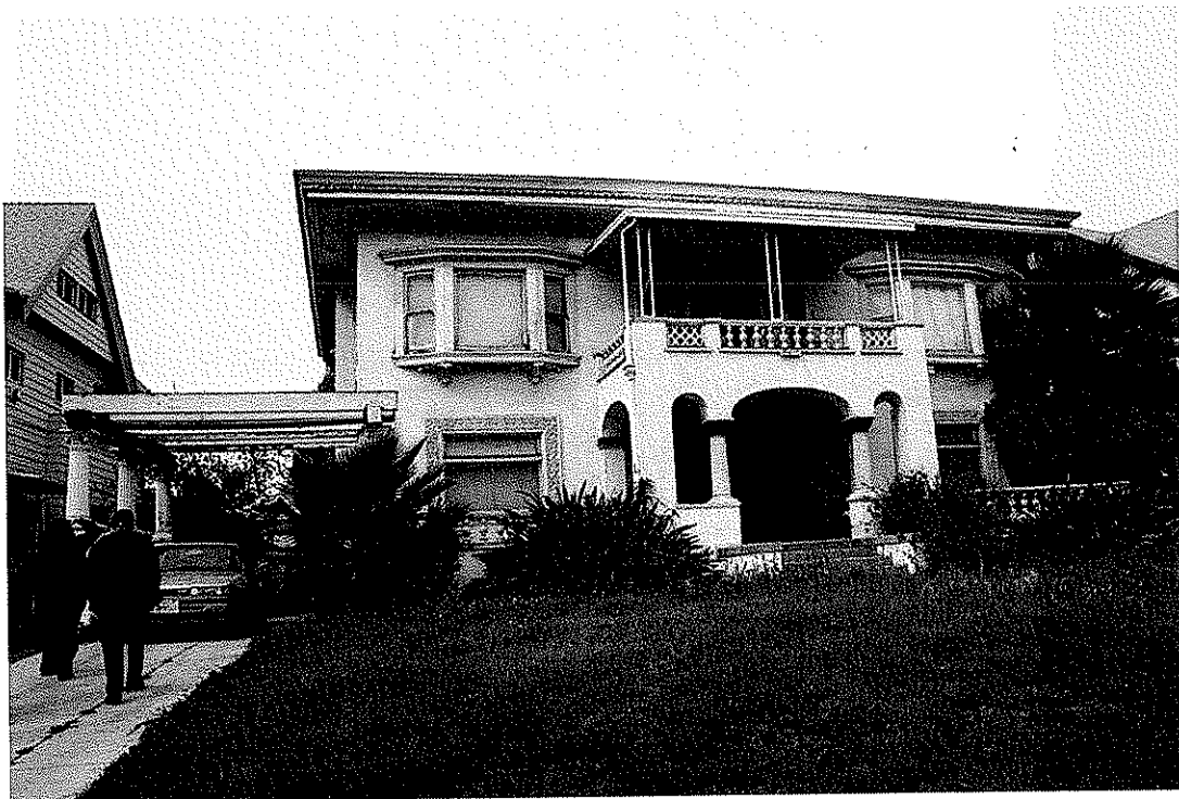
West façade, viewed to west.
