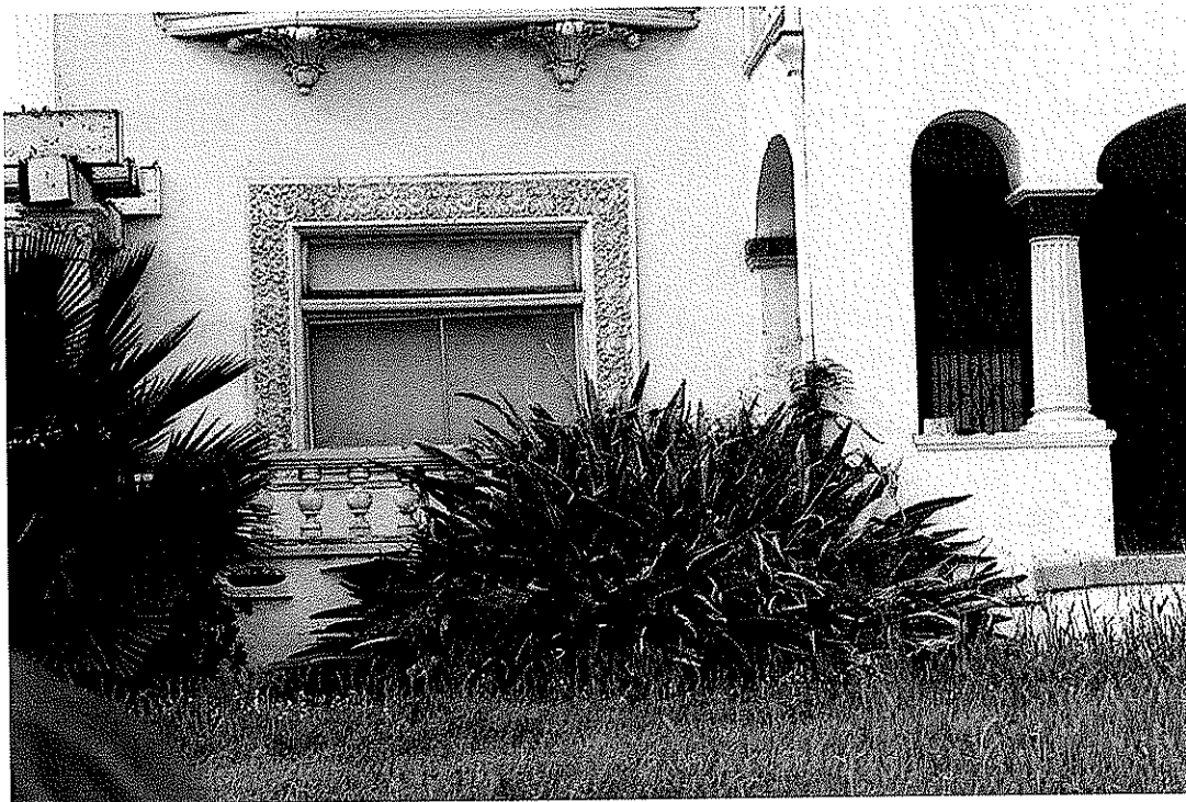
Details of west façade, viewed to west.
