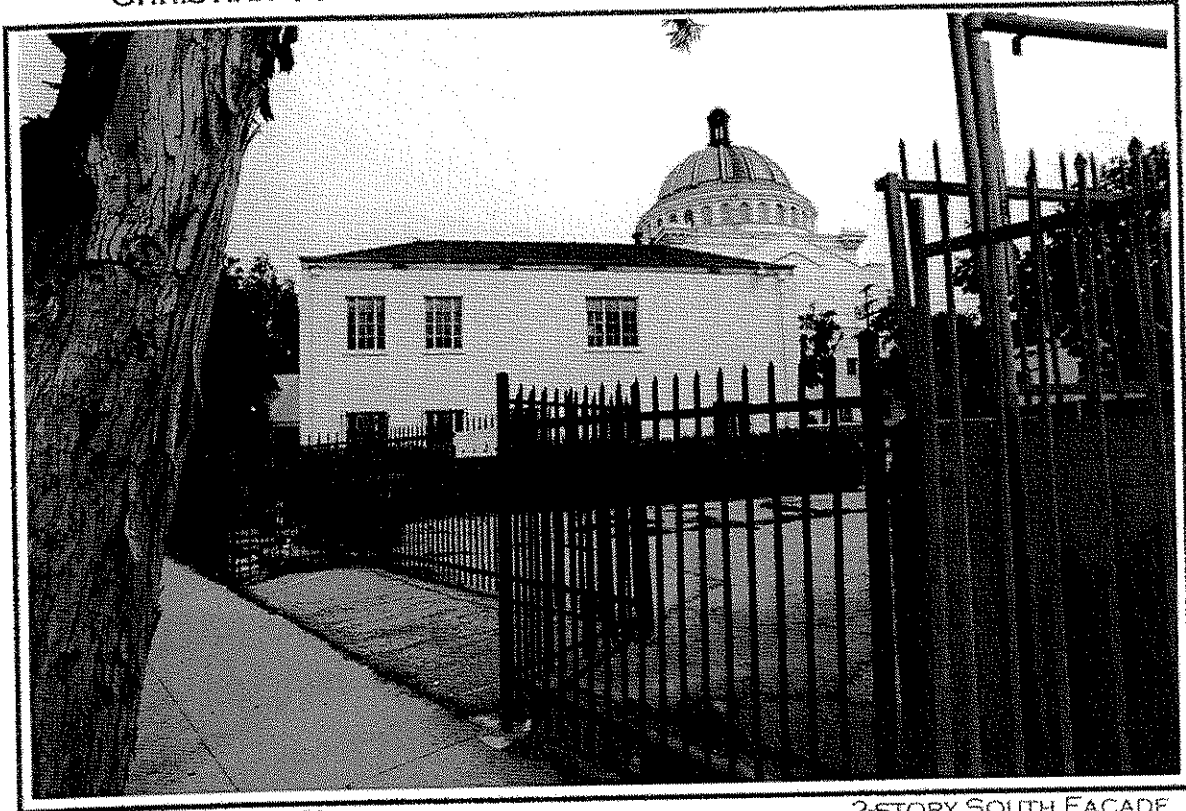
15). VIEW LOOKING NORTH
