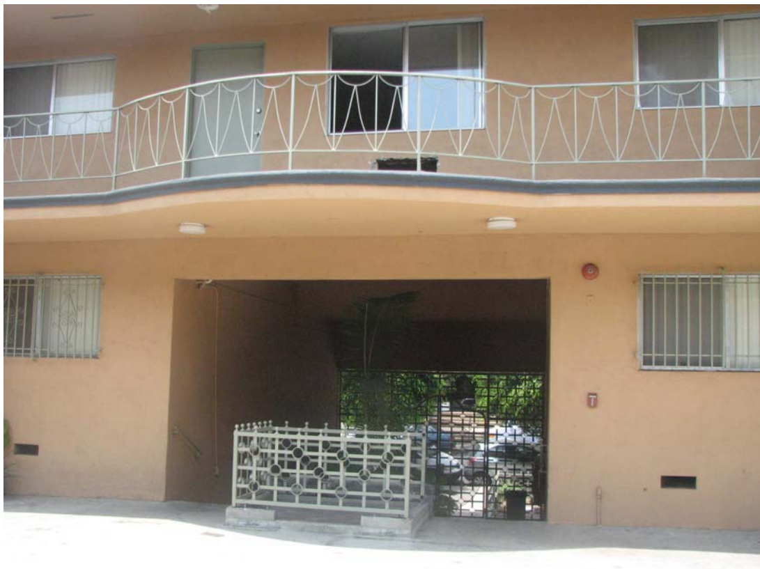
The Ardmore Wilshire, main entry from courtyard, 722 S. Ardmore Avenue, July 4, 2008 (photo by Charles J. Fisher)
