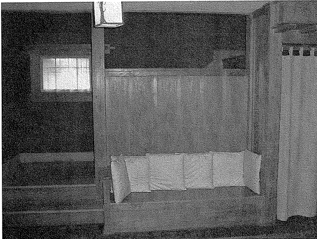
Stair landing and built-in bench viewed from east toward the west
