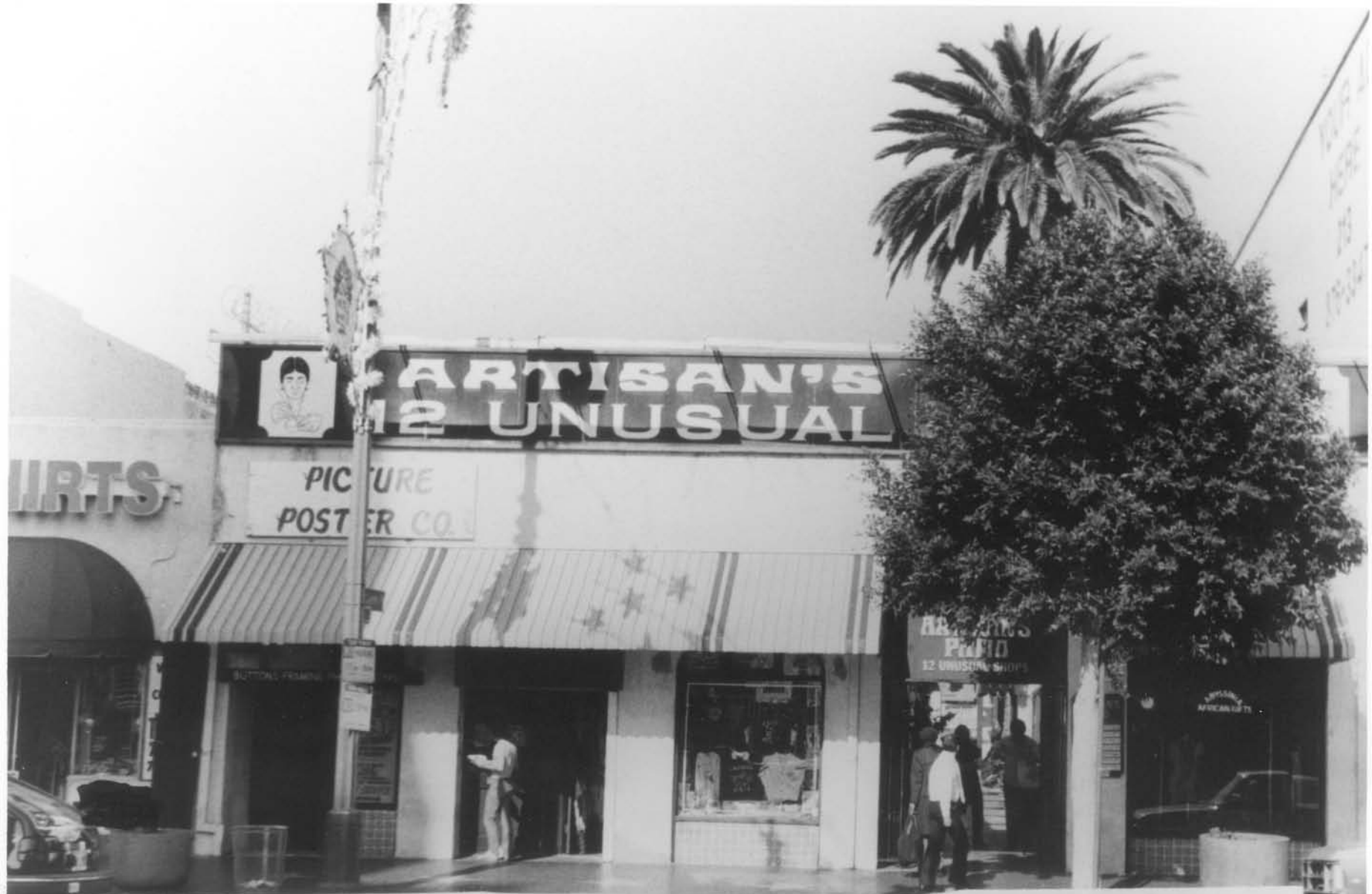
Photo of Hollywood Blvd. exterior of subject property. Overhead signs will be removed and replaced with more subdued signs similar to signs shown on architect's sketch enclosed. Entire site has just undergone a $100,000 seismic reinforcement job. This has resulted in shabby exteriors. Exterior will be restored with Spanish Style textured stucco coat, canvas awnings, and new paint also similar to architect's sketch.
