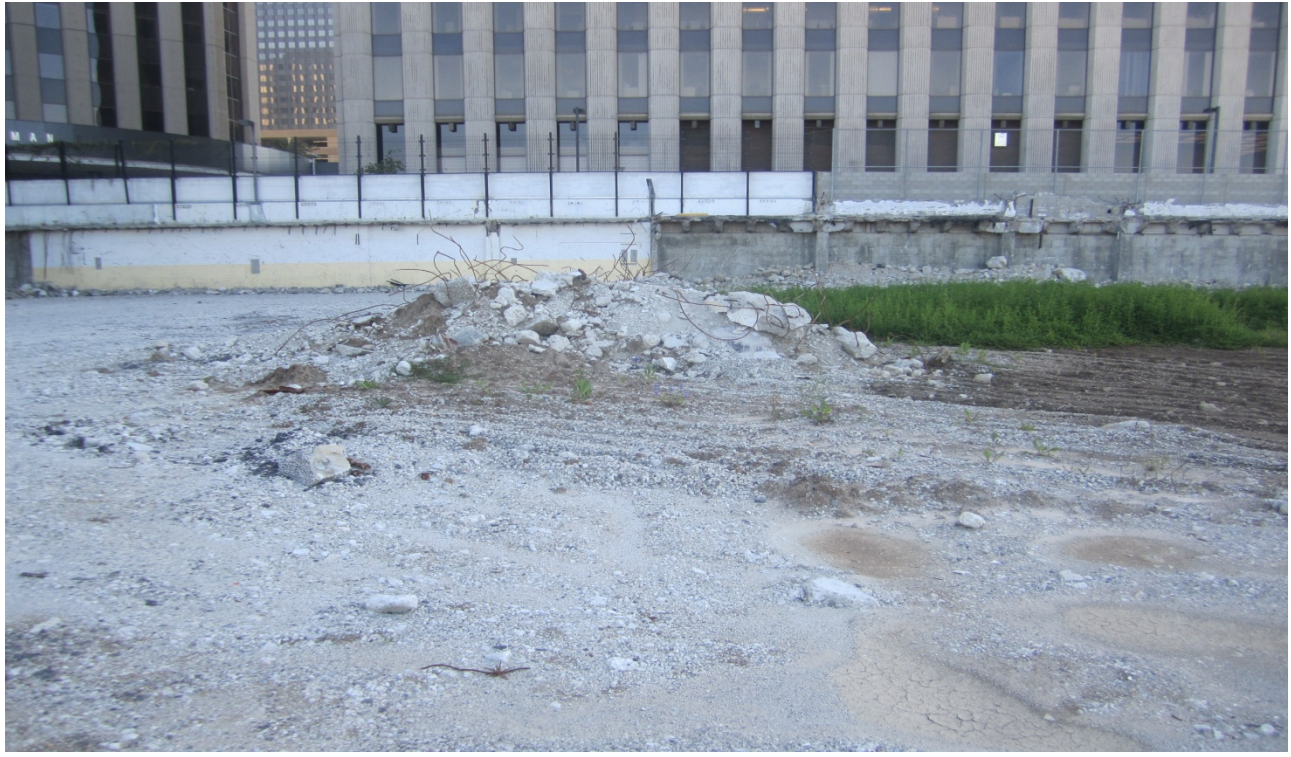
Photo 7: A small concrete pile located on the southwestern portion of the site.
