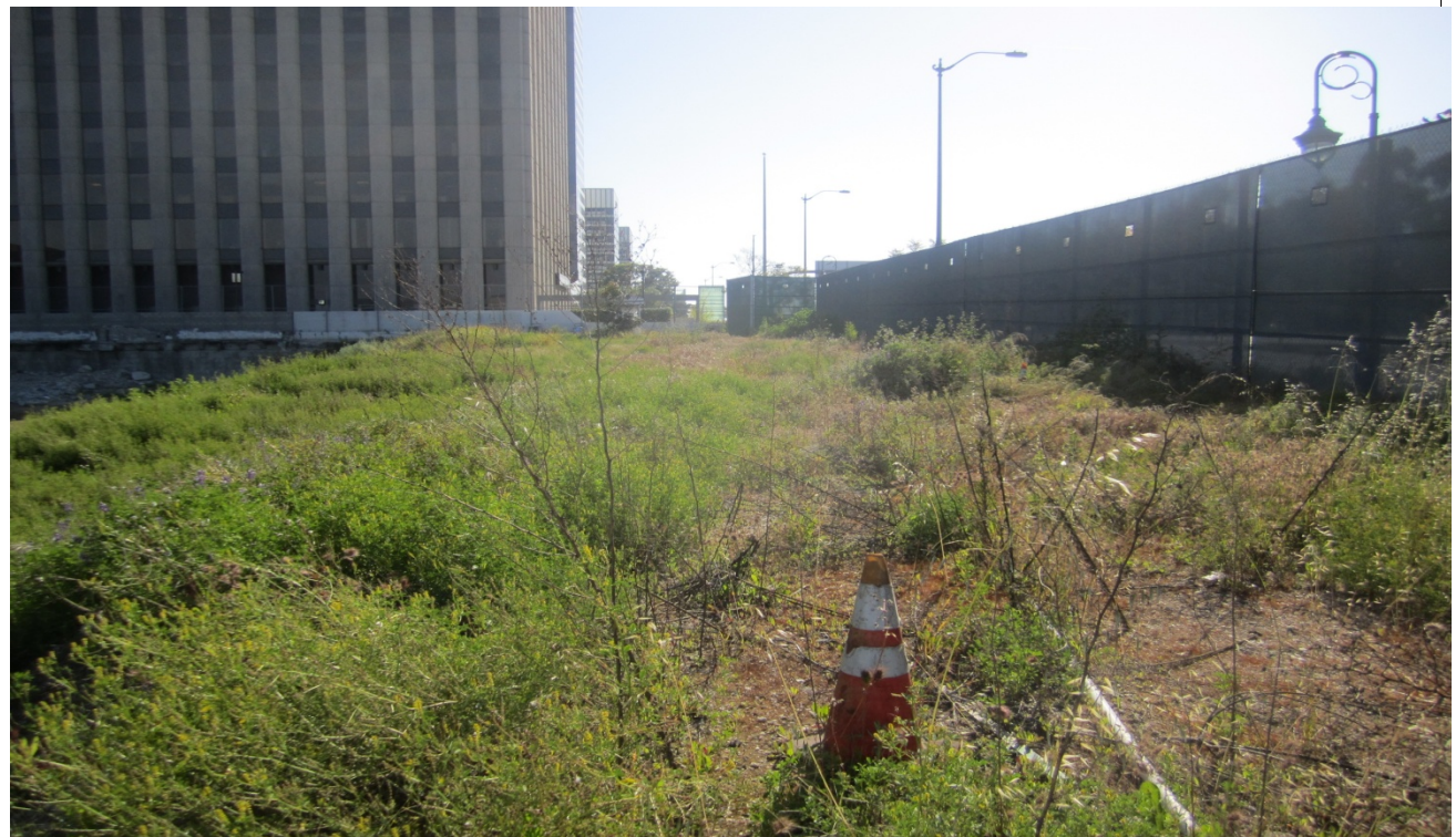
Photo 4: View of the northern site boundary, facing southwest.
