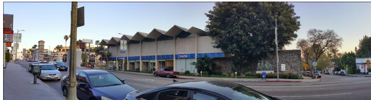
2A. VIEW FROM SUNSET BLVD. AND HAVENHURST DR.
