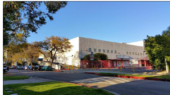
2D. VIEW FROM SOUTHWEST CORNER OF THE SITE
