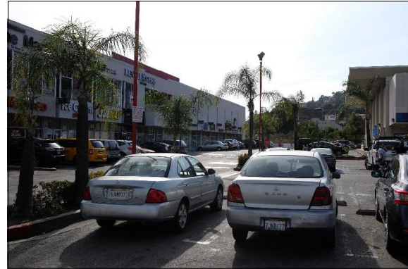
2E. EXISTING STRUCTURE, LOOKING WEST
