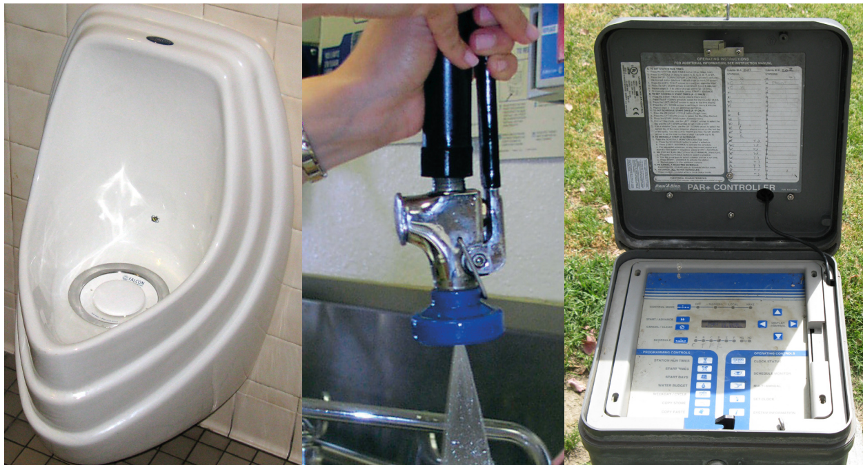
Water-saving opportunities have extended to the commercial and public sector with the introduction and support for new technologies such as the waterless urinal, pre-rinse spray head and centralized irrigation controller (pictured above left to right).
