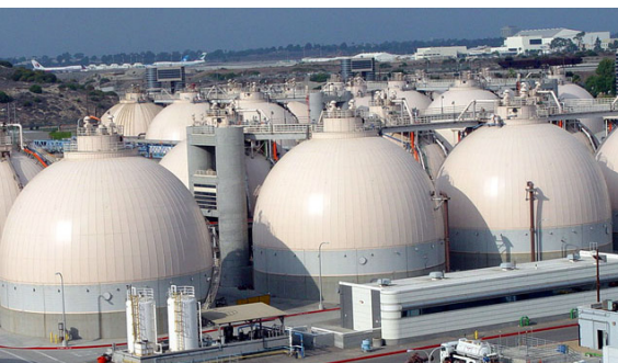
Egg-shaped Digesters at Hyperion
