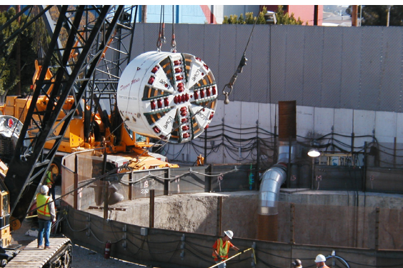
New Sewer Construction
