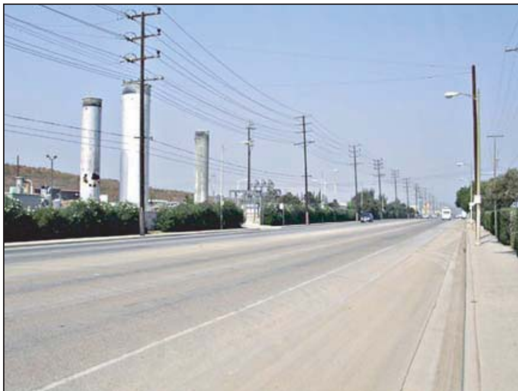
Photo B: View of existing landfill as seen from Glenoaks Boulevard looking towards its intersection with Sheldon Street.
