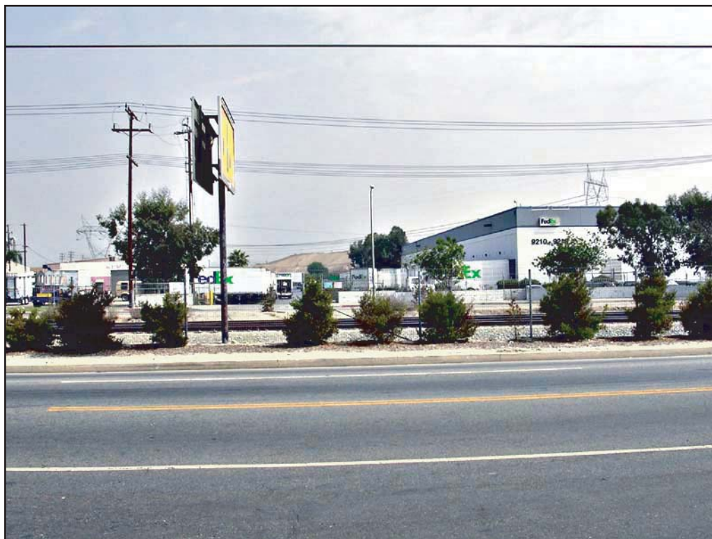
Photo B: View of the FedEx facility located on San Fernando.
