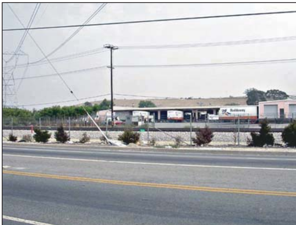
Photo D: View of the Bradley Landfill from San Fernando Road looking northeast.
