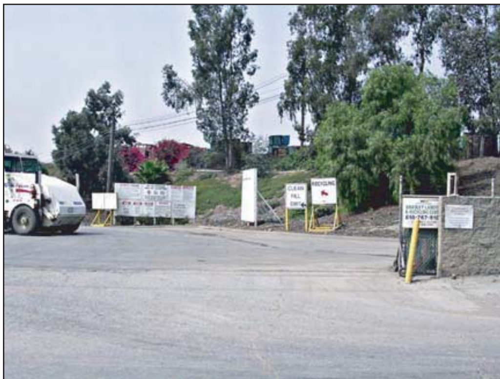
Photo F: View of the Bradley Landfill entrance looking west from Tujunga Avenue.
