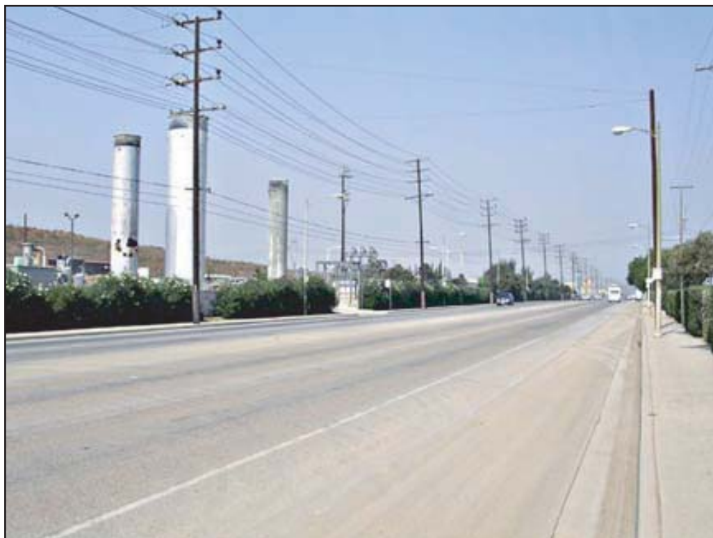
Photo J: View of Glenoaks Boulevard looking towards its intersection with Sheldon Street. The existing landfill is visible on the left.
