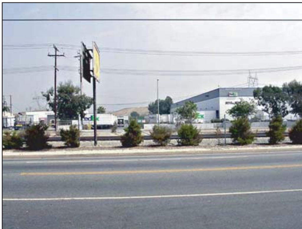
Photo N: View of the FedEx facility located on San Fernando Road. The Bradley Landfill is visible in the background.
