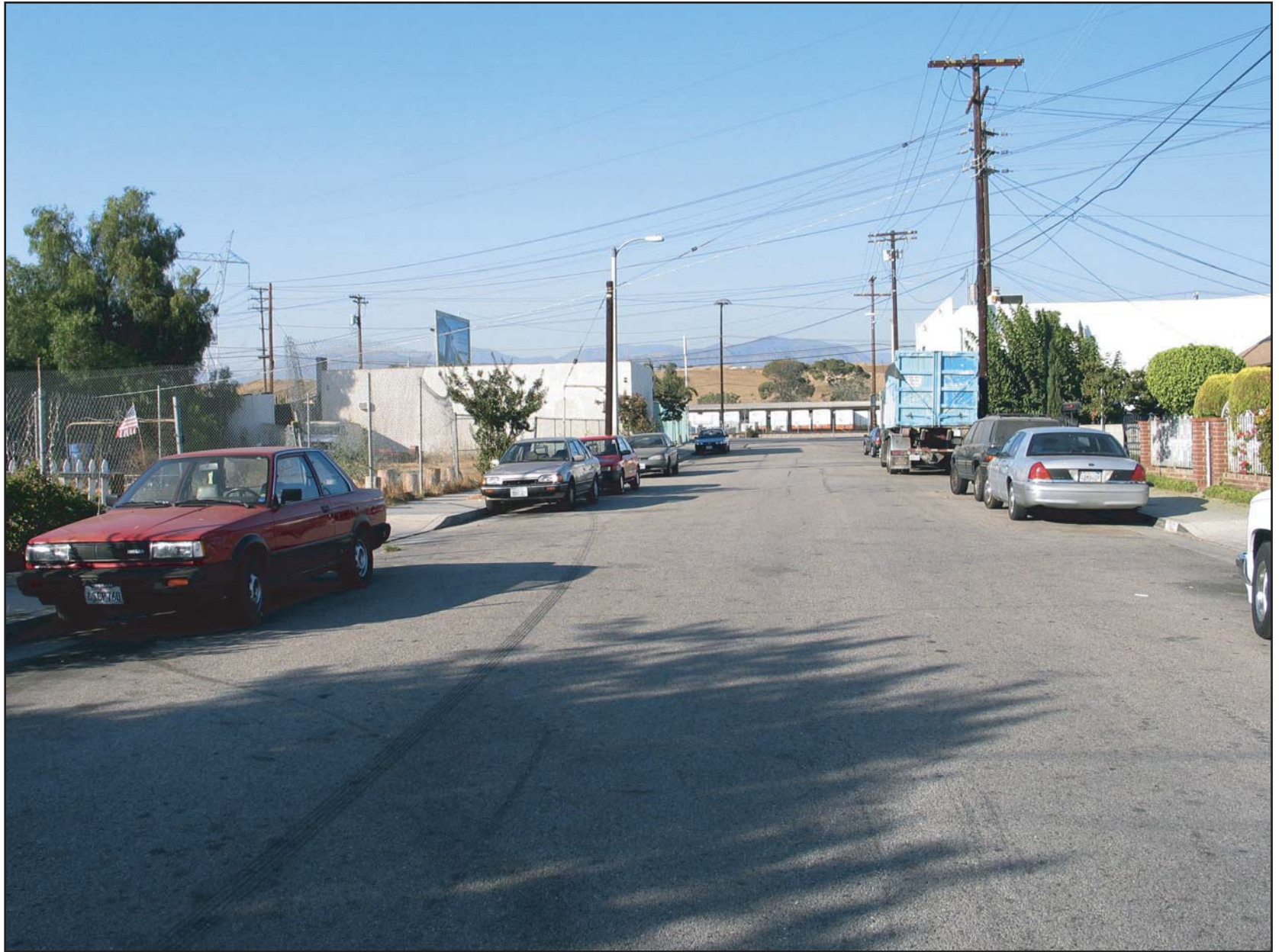
Photograph A: View of the existing Bradley Landfill as seen from Art Street.
