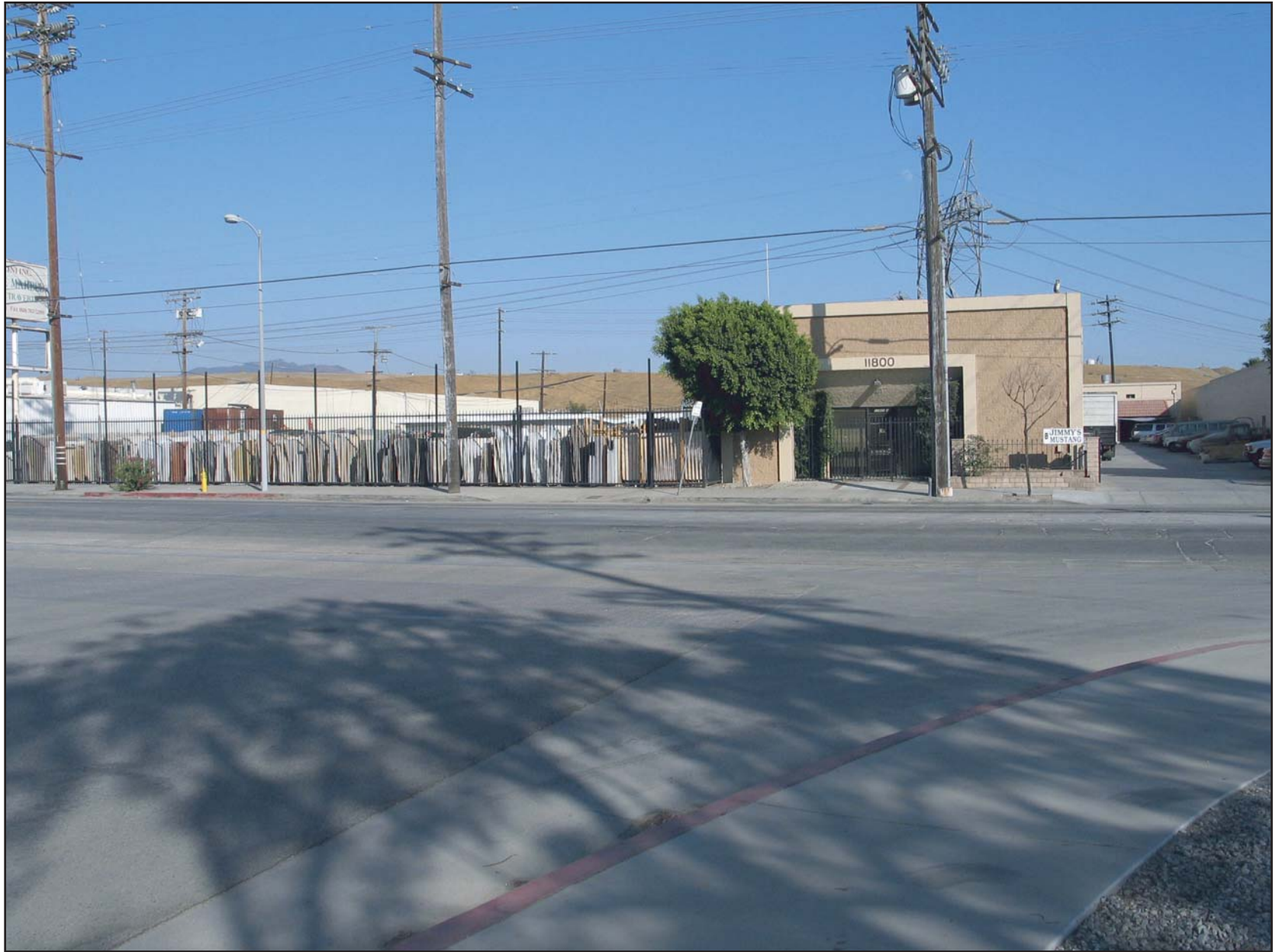
Photograph A: View of the existing Bradley Landfill as seen from Sheldon Street.
