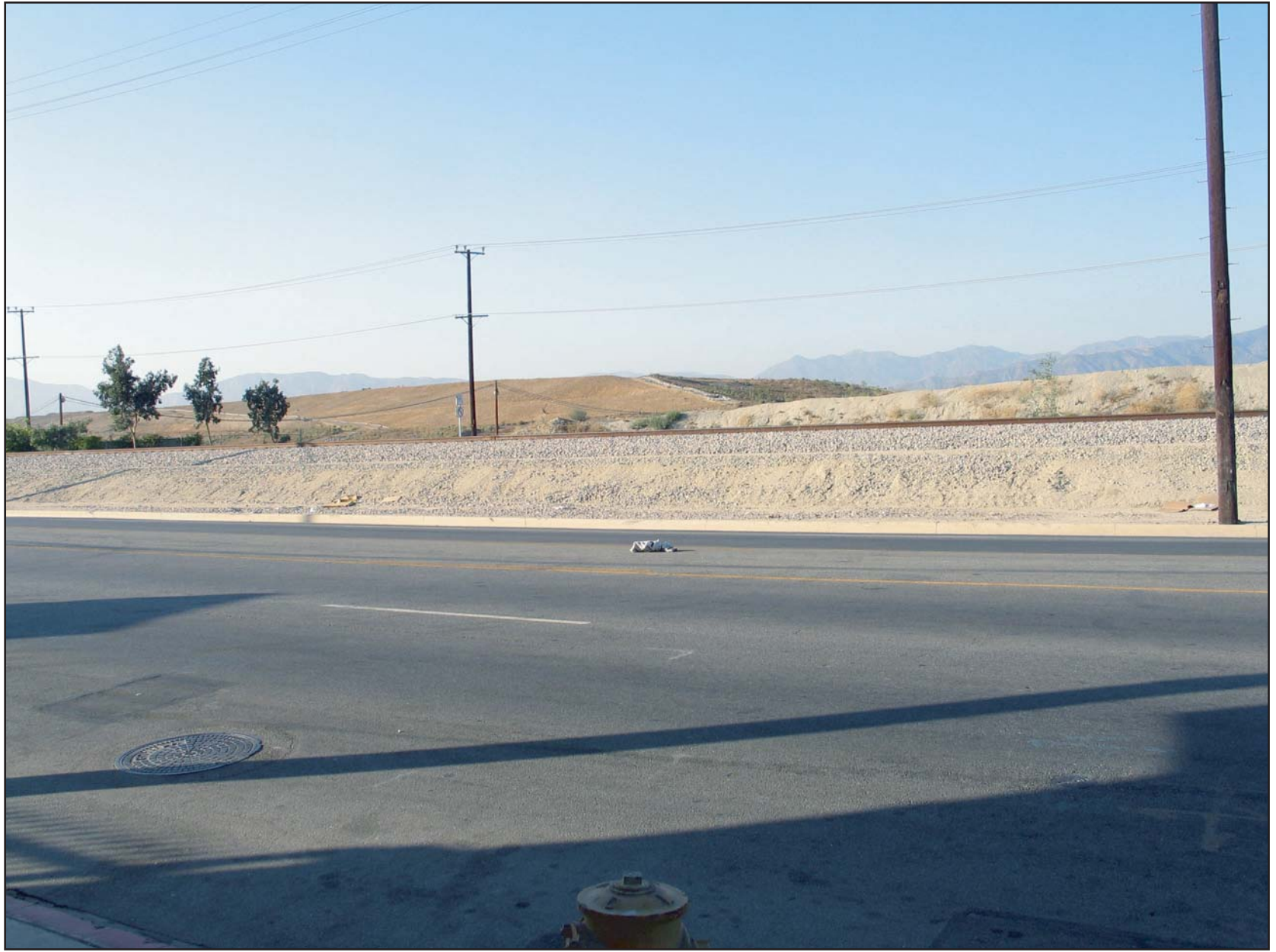
Photograph A: View of the existing Bradley Landfill as seen from San Fernando Road between Lankershim Boulevard and Tuxford Street.
