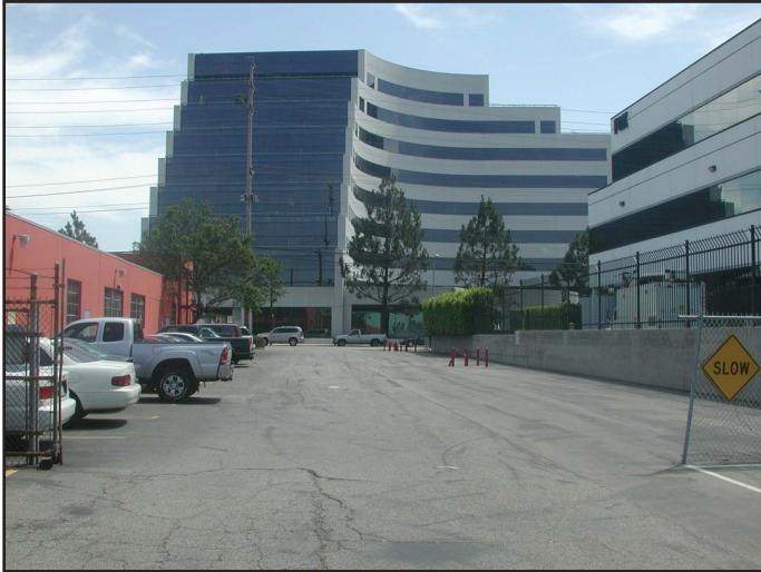
View 13: Looking northeast from the Bundy Drive entrance to the project site towards Bundy Drive and a high-rise office building. Commercial brick buildings on the project site are located to the north (left) and the Fox Studios building to the south (right).
