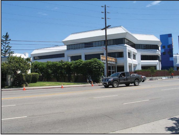
View 20: Looking northeast across Olympic Boulevard towards the Teledyne Controls building and the three-story Tribeca West building.
