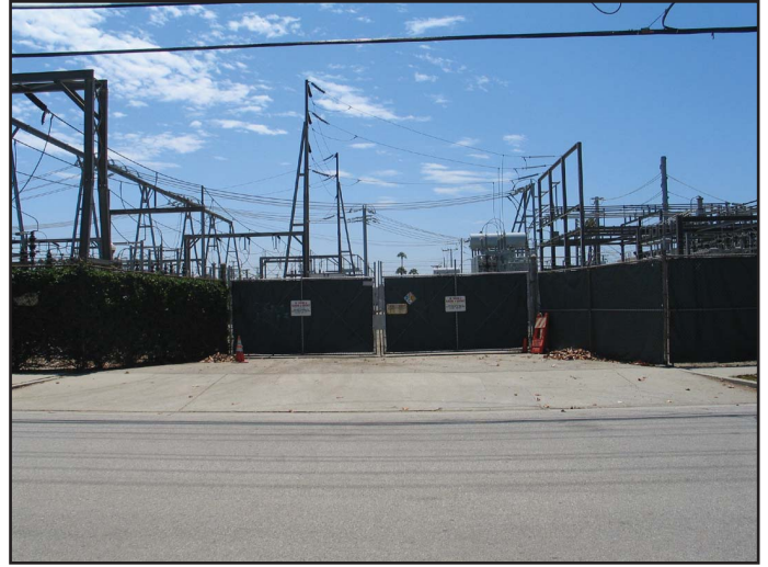
View 21: Looking southeast across Nebraska Avenue towards the LADWP Yard.
