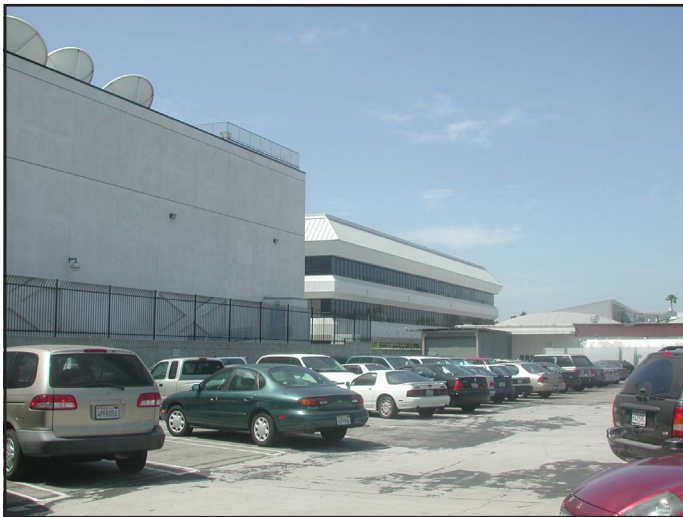
View 12: Looking southwest across the surface parking lot located in Parcel A, with the Fox Studios and Tribeca West buildings in the background. The Teledyne Controls building is also located in the background, to the north (right).
