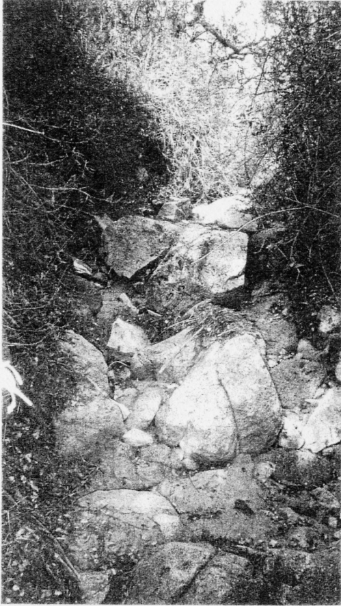
Photograph 12. Looking northeast up the main drainage.
