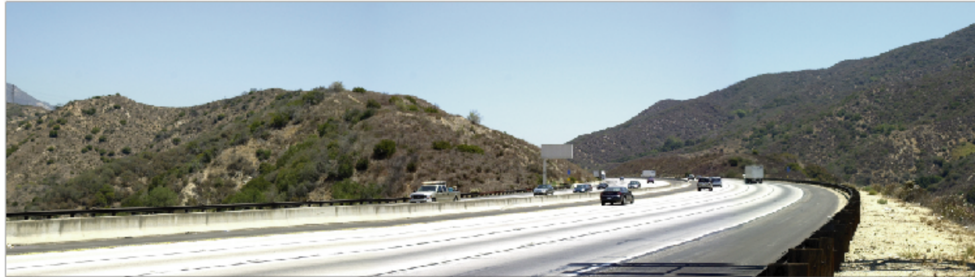
Existing view from the shoulders of Interstate 210 looking northeast toward the proposed Development Area A.
