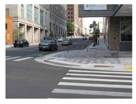
This corner has curb extensions, directional ramps and special paving for enhanced visibility and identity.
