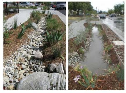
1. Parkways at sidewalk level with a swale or depression to collect and infiltrate sidewalk runoff. This example on Elmer Avenue in Sun Valley also infiltrates street runoff. (photo source: Council for Watershed Health)
