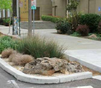
4. Curb extensions at street level with curbs. In this example runoff flowing along the gutter is directed into the curb extension swale where it can be absorbed into an "infiltration gallery" beneath the surface; in a heavy rain, excess runoff flows back into the gutter and into the existing storm drain system. (photo source: land8.com)
