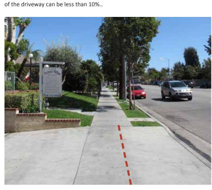
Where the sidewalk is at least 11' wide and the parkway is at least 5.5' wide, the sloped area of the driveway can align with the parkway. In this portion of Pico Blvd., the sidewalk is 15' wide and the parkway is wider than 5.5', so the slope
