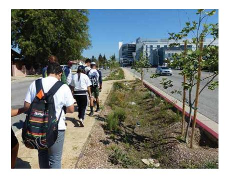
5. Medians along the slope of the roadway crown can collect runoff directly through breaks in the median curb. In this example on Woodman Avenue in Sun Valley, Los Angeles, the median divides the primary roadway (right side) from a residential frontage road (left side) and openings in the curb on the right side.
