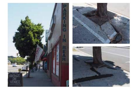
As these photos show, some already small tree wells have been filled with asphalt. Because the tree wells are so small, concrete is sometimes uplifted.
