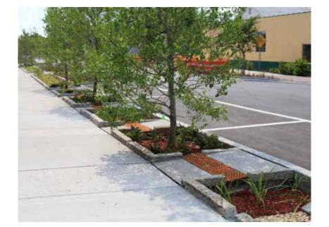
2. Tree wells at sidewalk with depressed soil level and curb breaks to collect street runoff are connected to function as a continuous infiltration basin. Curbs are often required where the soil level is lower than the sidewalk, as shown here. Overflow is released back into the street at the end of the connected tree wells.(photo source: Blue-Green Building.org)
