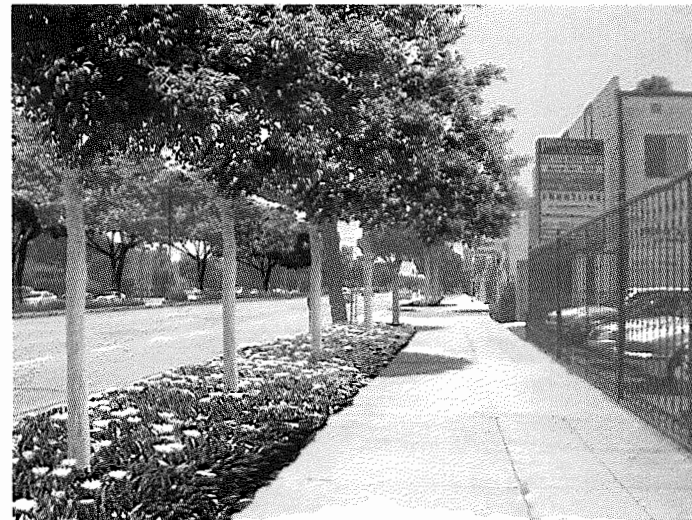
PROPOSED STORMWATER PARKWAYS replace existing areas of paving to create a more vibrant setting along Venice Boulevard. In more commercial areas along Venice Boulevard, porous paving will be used instead of planting beds to further reduce stormwater runoff. Reengineering the soil will assist drainage as well.
