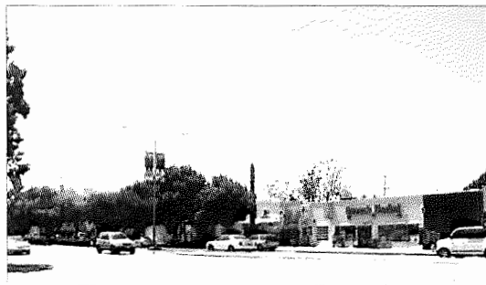
EXISTING STREETScape OF RESIDENTIAL DISTRICT
