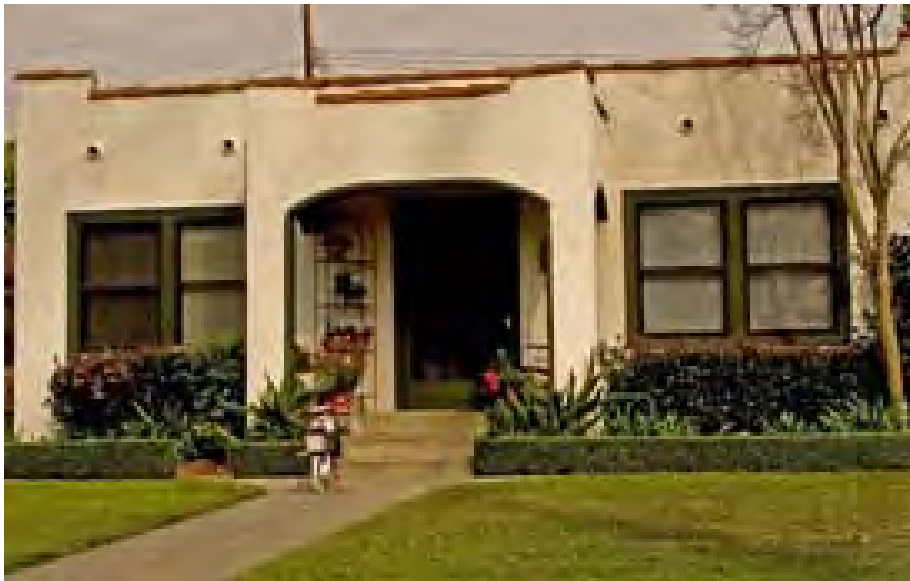
Figure 10. Residence at 1105 E. Whiting Avenue, Fullerton ( http://www.fullertonheritage.org/Resources/archstyles/pueblo.htm , accessed 12/17/13)
