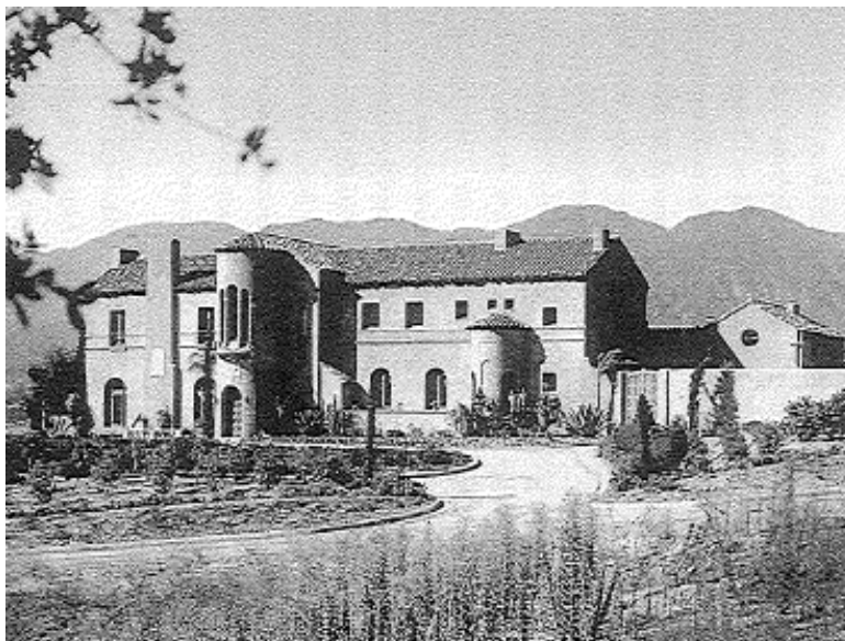
Figure 1. William P. Hanson House, by Henry Harwood Hewitt, 1920 (Sam Watters, "William P. Hanson House, Flintridge," Houses of Los Angeles , Volume 2, Acanthus Press, 2007, pp. 40 and 45)
