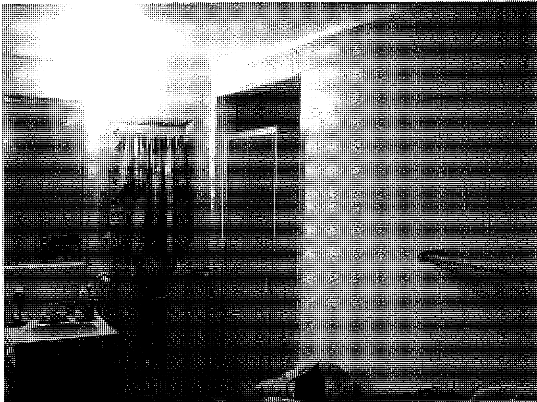
Elchar Residence, bathroom walls, 1401 N. Hobart Boulevard, October 4, 2010
