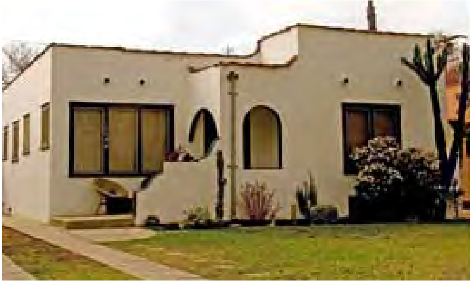
Figure 11. Residence at 1120 E. Whiting Avenue, Fullerton ( http://www.fullertonheritage.org/Resources/archstyles/pueblo.htm , accessed 12/17/13)
