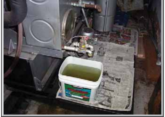
View of the dry cleaning equipment.
