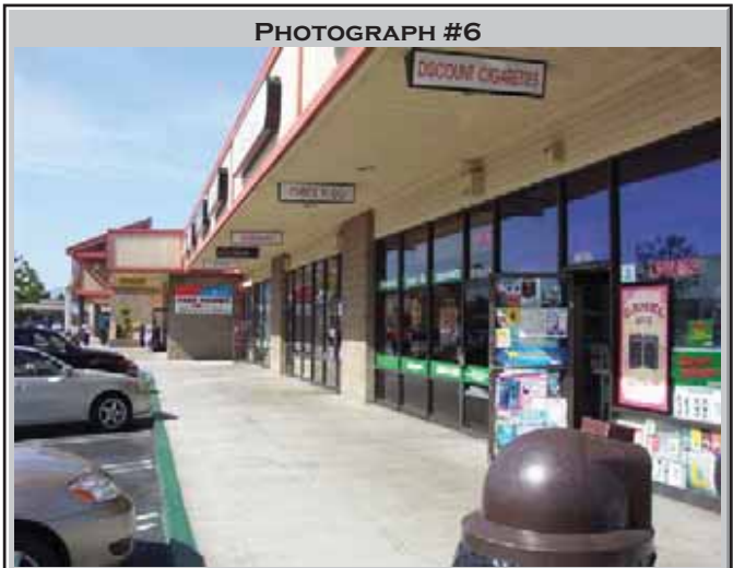
Exterior view of the tenant spaces.
