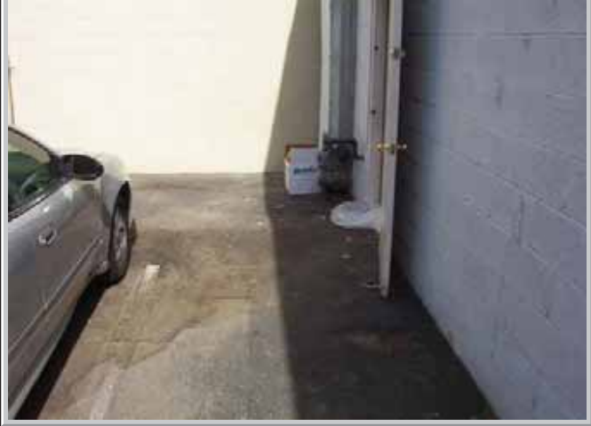
View of the rear door at the Victory Plaza Cleaners.
