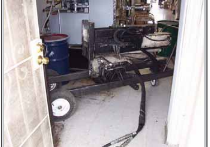
View of drilling interior Boring #1 at the Victory Plaza Cleaners.
