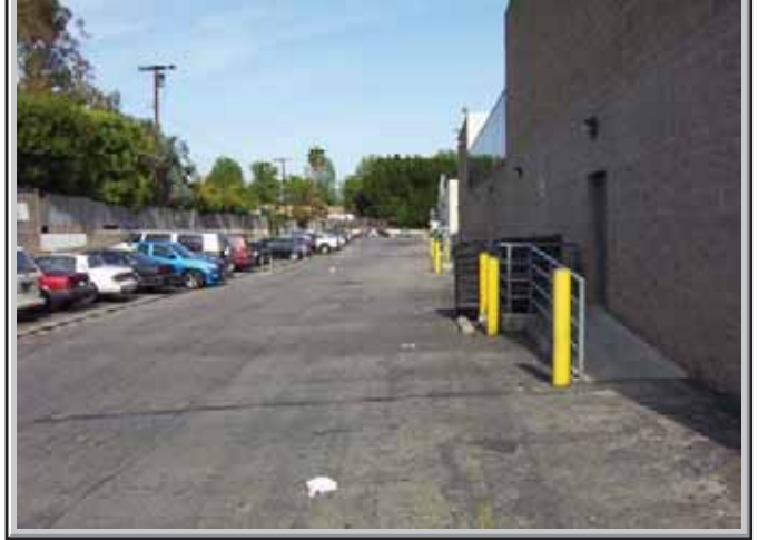
Exterior view of the rear of the subject property building.
