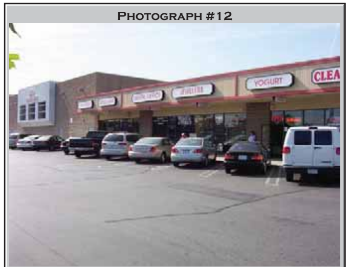
Exterior view of the tenant spaces.
