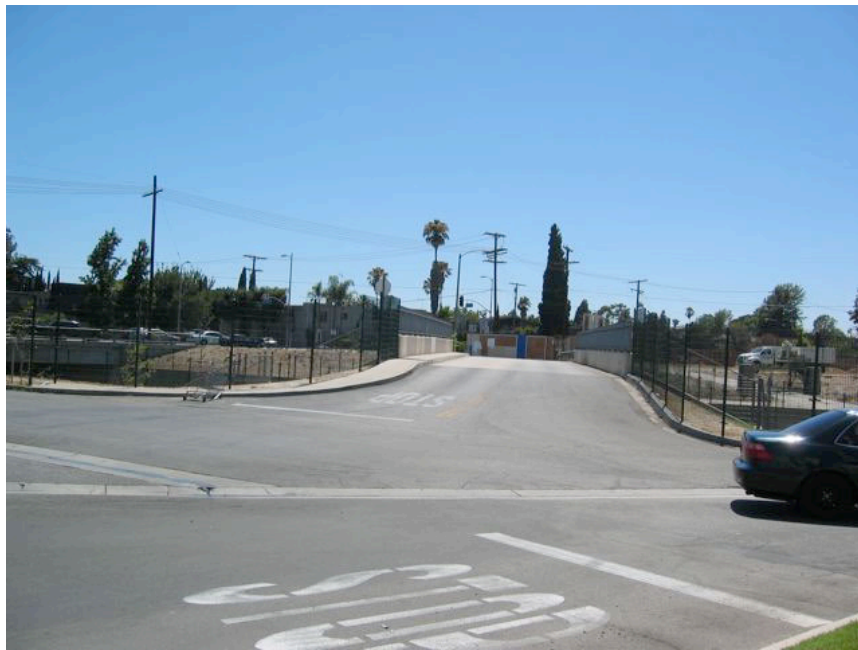
Figure III-11: View West from Ethel Avenue Entrance across Tujunga Wash
