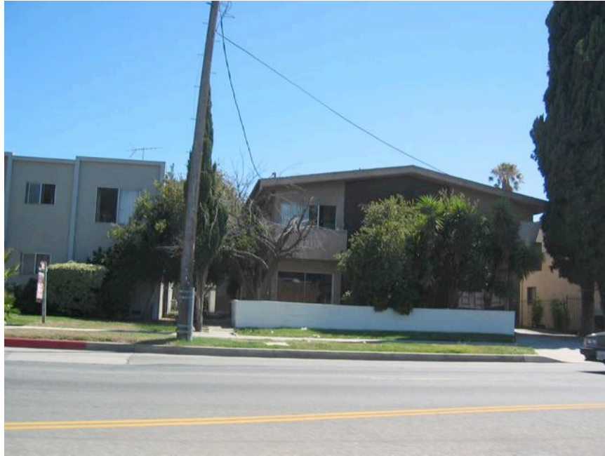
Figure III-8: View of Multi-Family Housing Southwest of Site across Victory Boulevard, West of Ethel Avenue
