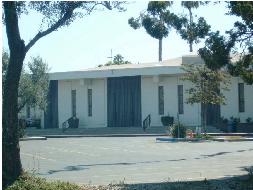
Figure IV.A-5: View of Church located on Add Area looking northeast from Victory Boulevard
