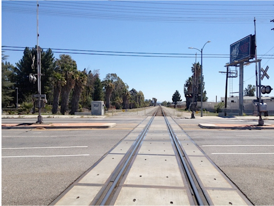
Figure III.A-1: View Southeast along Southern Pacific Railroad Right-of-Way along the Southern Boundary of the Project Site
