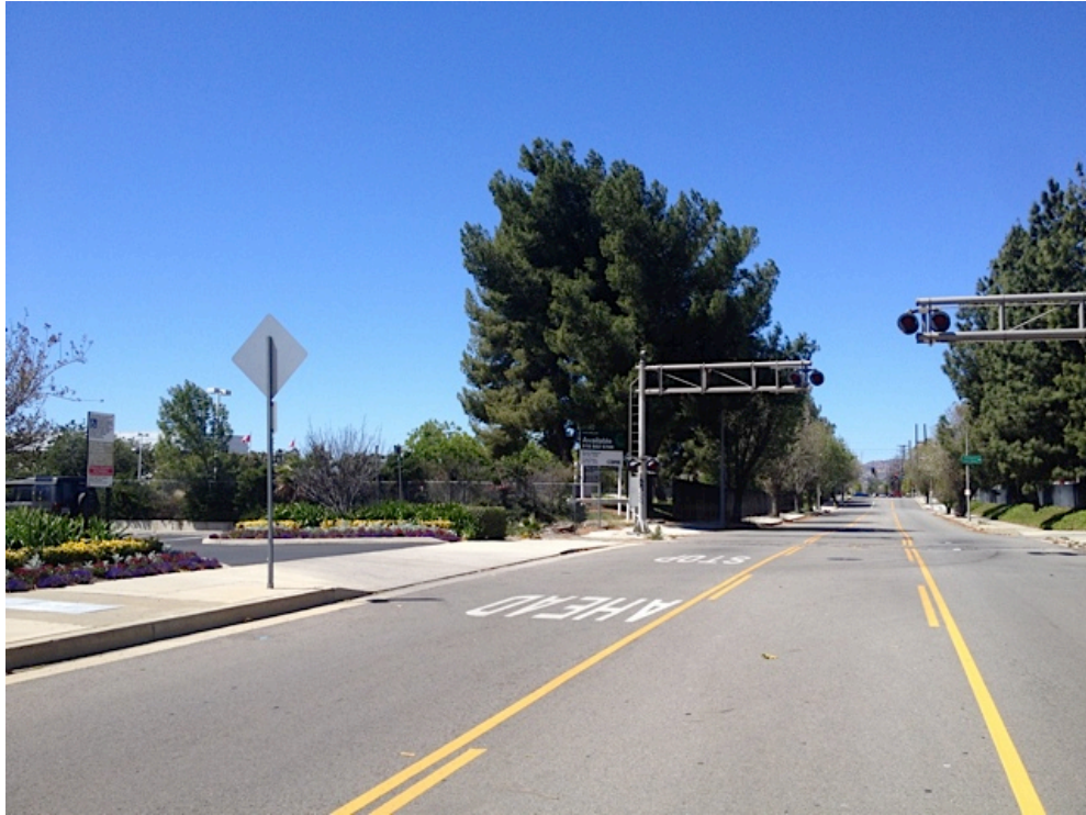
Figure III.A-12: Existing Conditions Viewpoint # 4 - View looking West along Prairie Street (View of the Northern Project Site Boundary)
