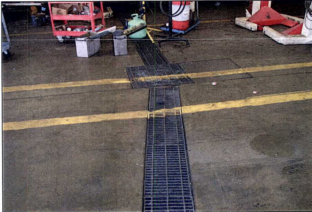
Photograph 15: Trenches and clarifier located in eastern portion of West Wing.
