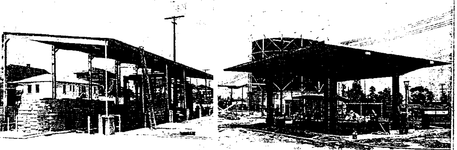
AUTOMATIC BUS WASHER building at west end of lot, with silhouetted outline of bus washing machine visible toward end of building. Stacks of concrete blocks on floor are for building the west wall of the shed. Left corner of picture shows wall partially built.
