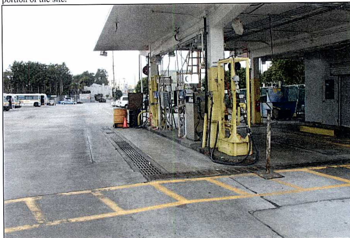
Photograph 6: Fuel pump island located on southeastern portion of site.
