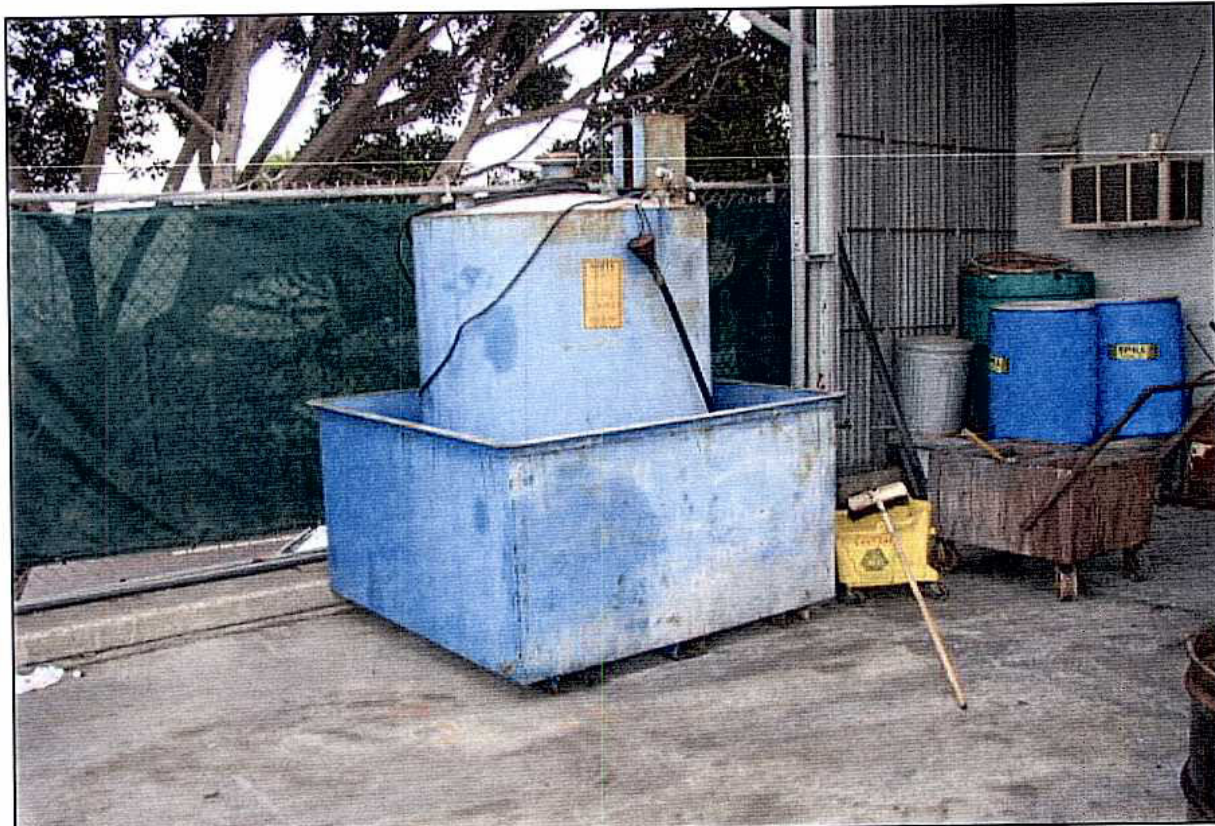
Photograph 17: Container of used anti-freeze/coolant on secondary containment platform.
