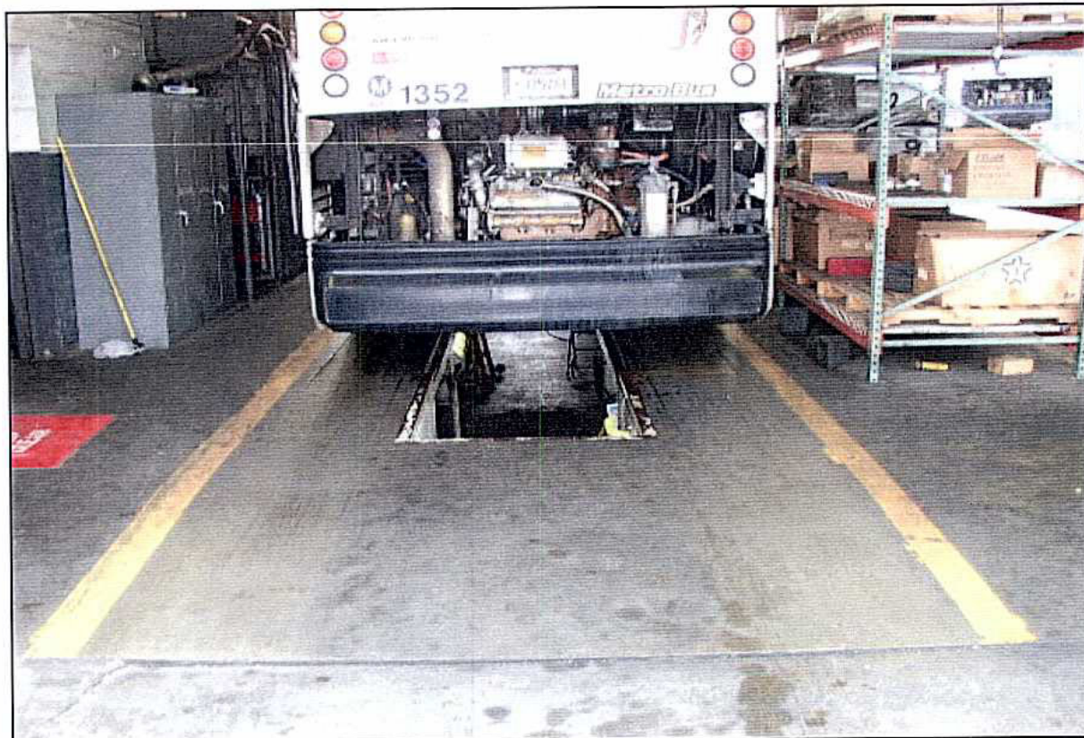
Photograph 11: Inspection/repair pit in South Wing.
