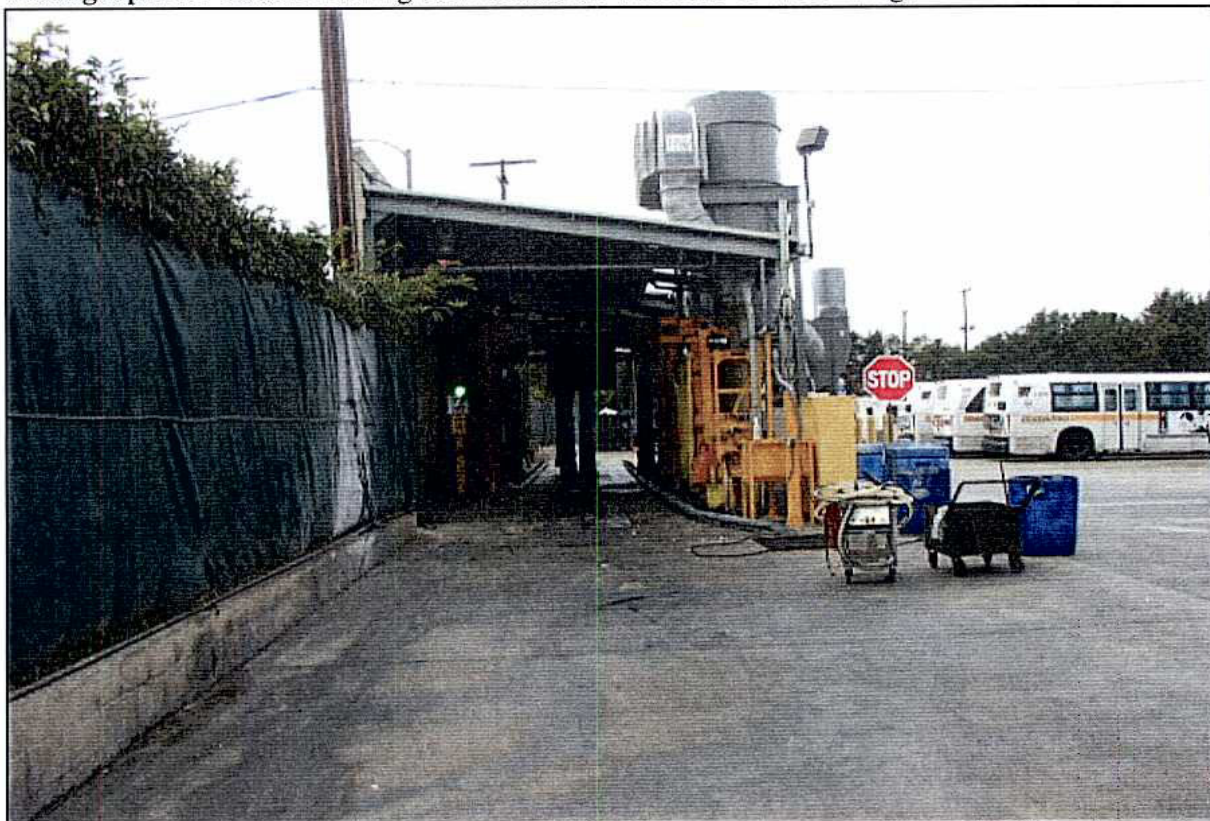
Photograph 14: Entrance to bus wash rack located on western edge of site. View is to the north.
