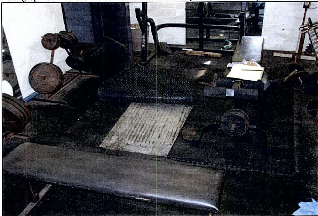
Photograph 16: Steel plate covering clarifier in the former battery room (now used as an employee weight room/gym).
