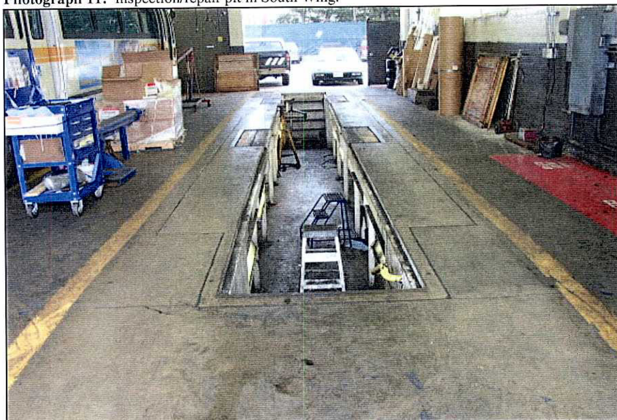
Photograph 12: Inspection/repair pit located in western portion of West Wing.
