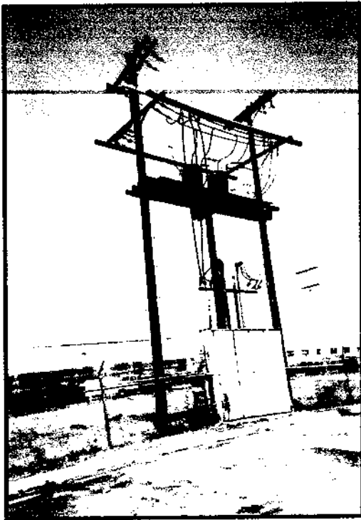
Pole-Mounted Electric Transformer, Adjacent to Western Boundary, Subject Site
