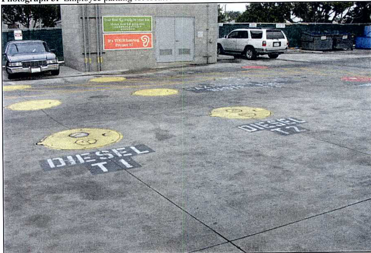
Photograph 4: USTs T-1 to T-4 located adjacent to fuel pump room on eastern portion of the site.
