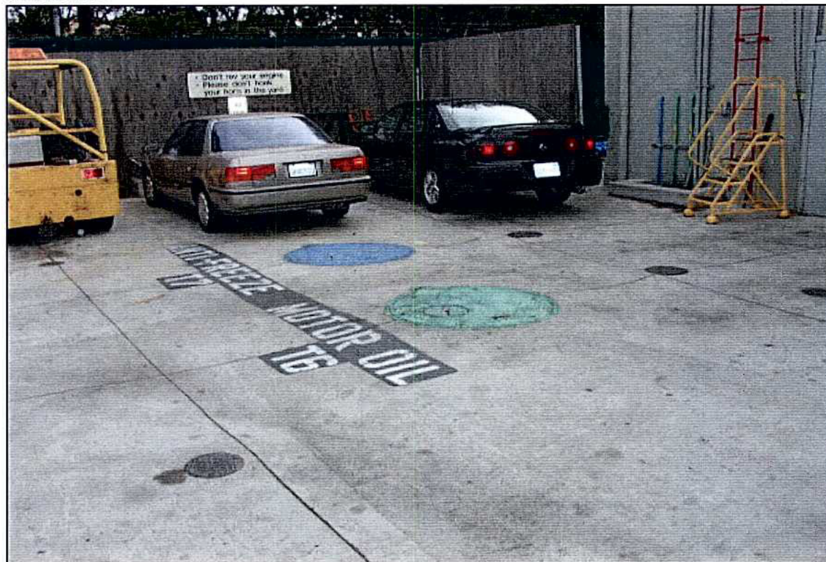
Photograph 8: Tank T-6 (motor oil UST) and T-7 (anti-freeze/coolant) located near southeast corner of South Wing.
