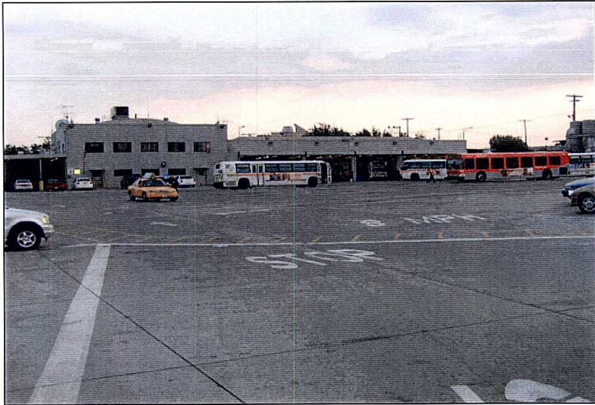
Photograph 1: Bus parking area and office/maintenance building. View is to the south-southwest.
