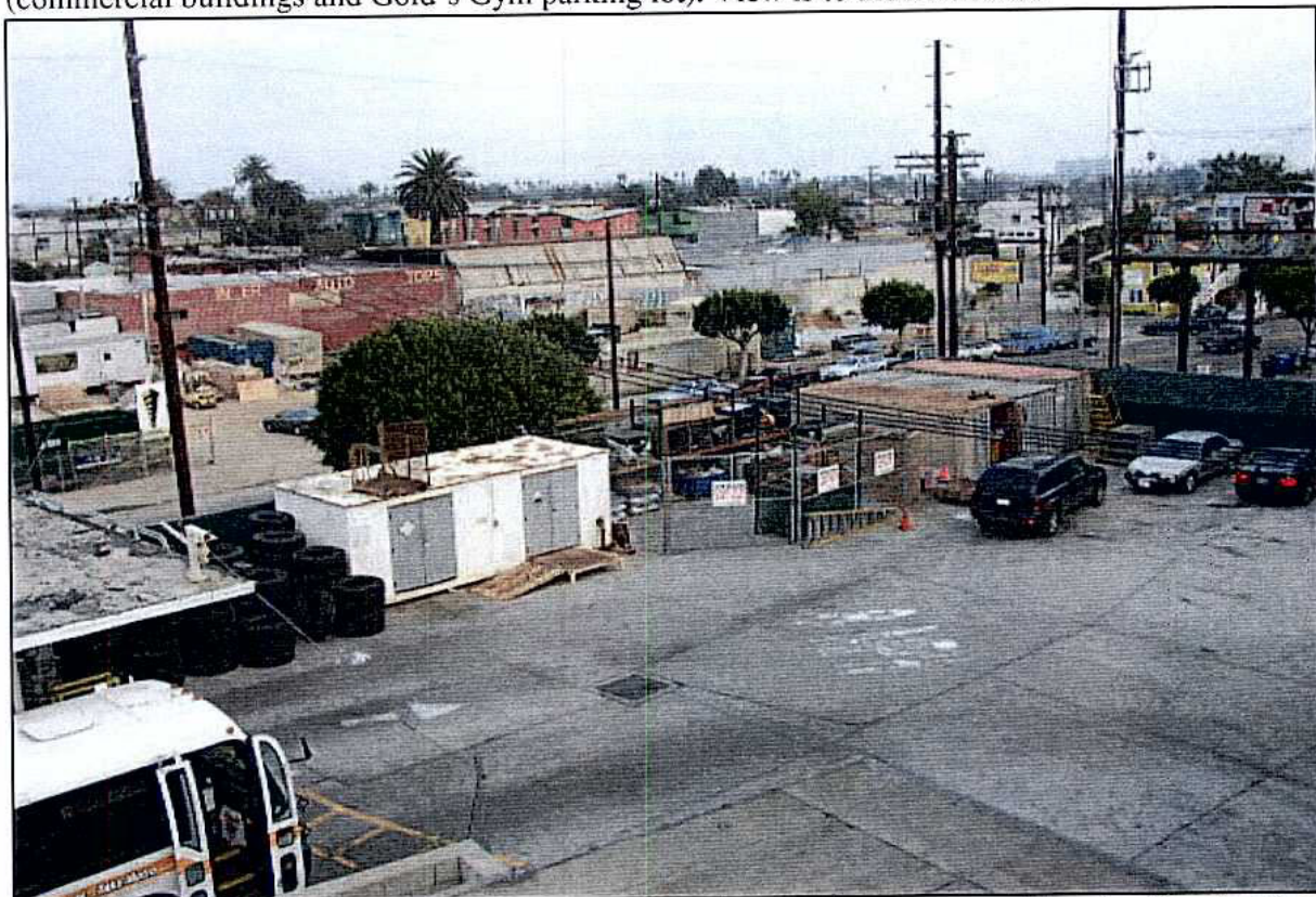
Photograph 20: Storage containers and storage yard on southeast corner of the site. Construction staging yard and commercial buildings on opposite side of Main Street in background. View is to the southeast.
