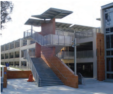
Solar panels on top of parking structure
