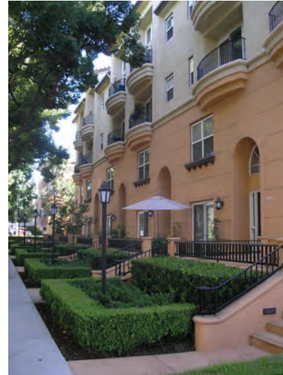
Example of townhome development in an urban neighborhood
