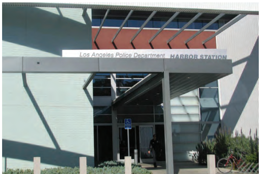
Los Angeles Police Department Harbor station, serving San Pedro
