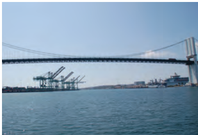
Vincent Thomas Bridge
