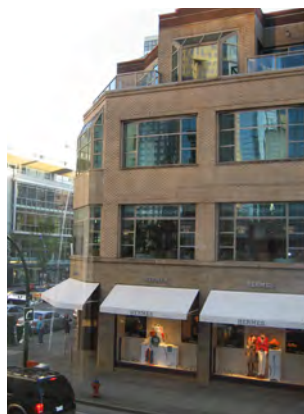
Guideline 2b example. This structure is stepped back above the 3rd story providing a variation in building mass.
